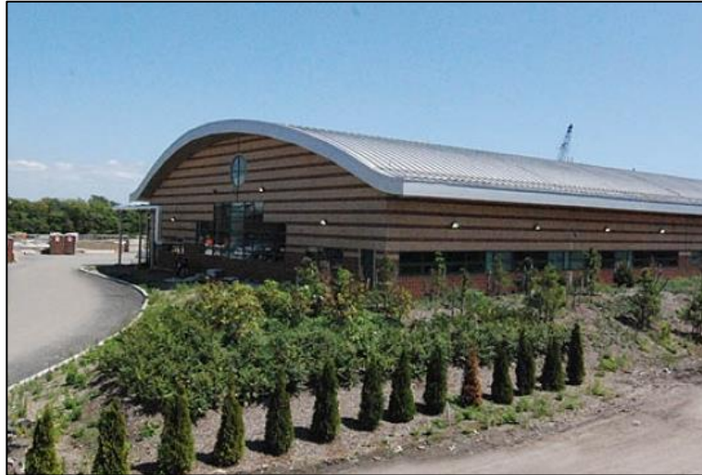
Figure 4-1: Paerdegat Basin CSO Facility
