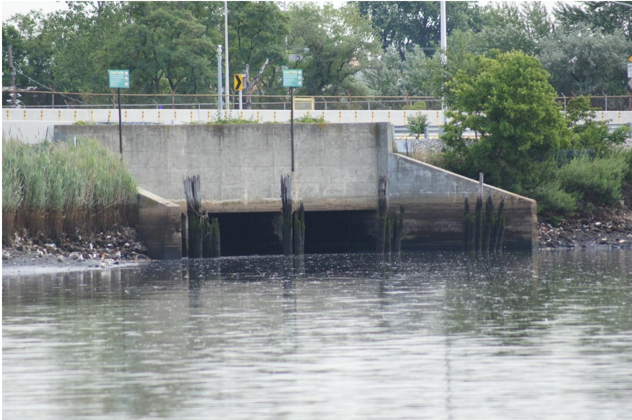
Figure 5. Bergen Basin Shoreline (Armored banks and Headwall for JAM-003/003A)
