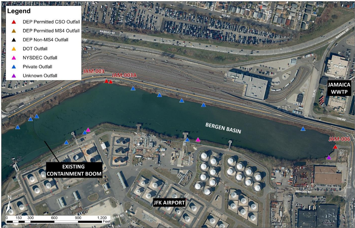
Figure 4. Bergen Basin Shoreline
