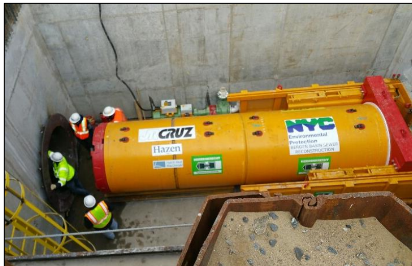
Figure 4-4: Microtunneling of New Parallel Sewer
