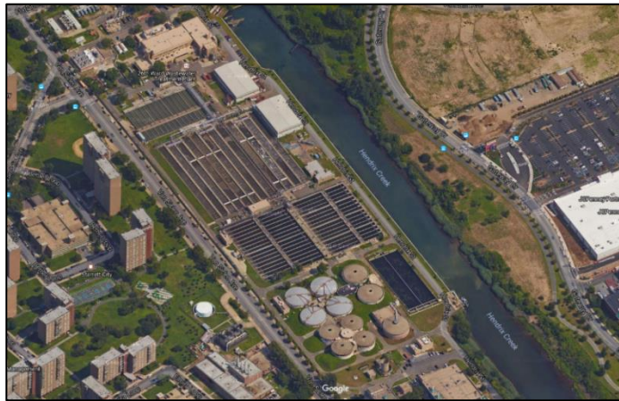
Figure 4-5: 26th Ward WWTP Wet Weather Stabilization
