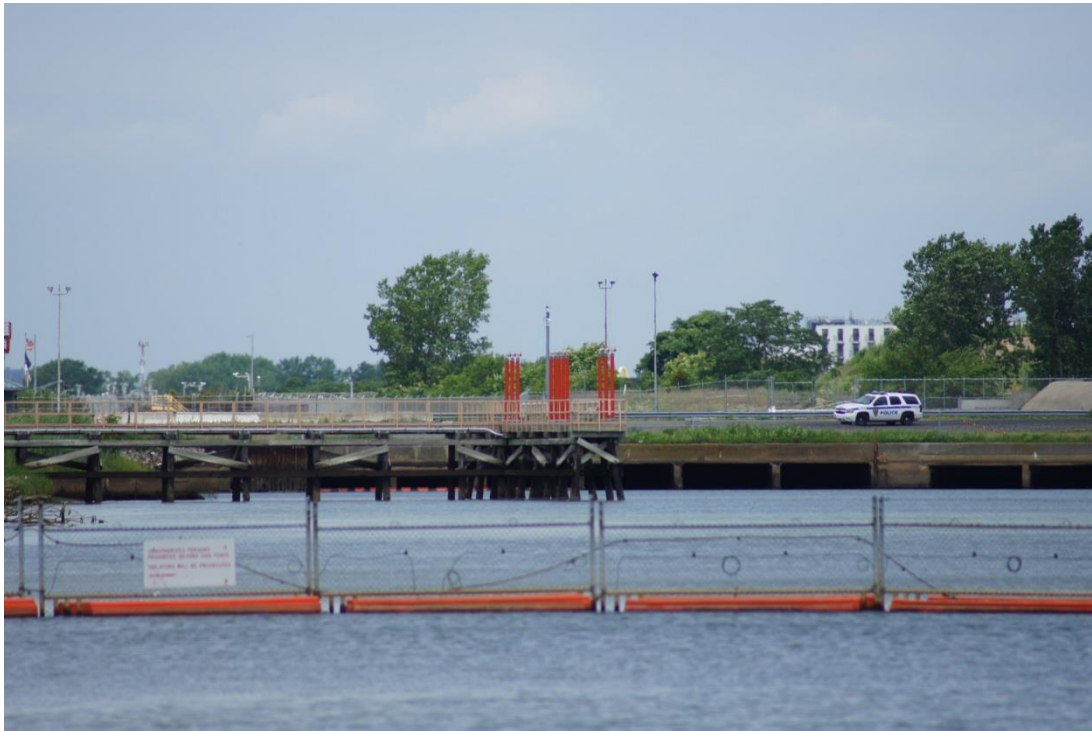
Figure 2-53. Photograph of Head End of Thurston Basin, showing Fence Restricting Access
