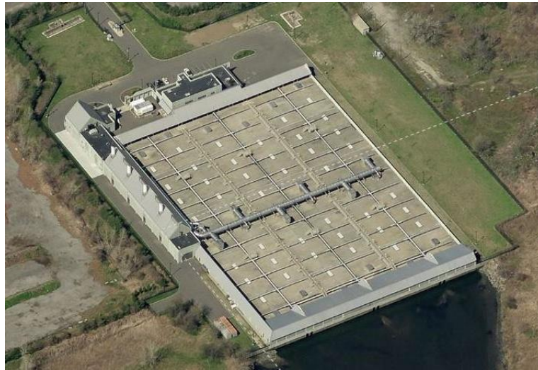
Figure 4-2: Spring Creek AWWTP
