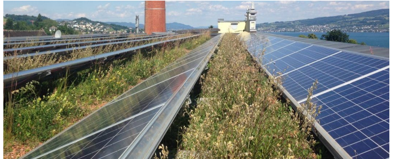
Bio-Solar Roof with Integrated Ballasts [2]
