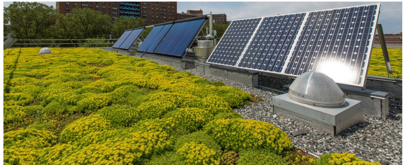
Bio-Solar Roof with Separate Ballast [3]
