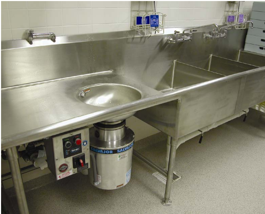
Image 1.1—An example of a commercial food waste disposer. This study looks at the effects of allowing restaurants and other food service establishments to use these units throughout New York City.
