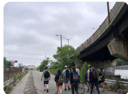
Existing: Exterior Street at Depot Place
