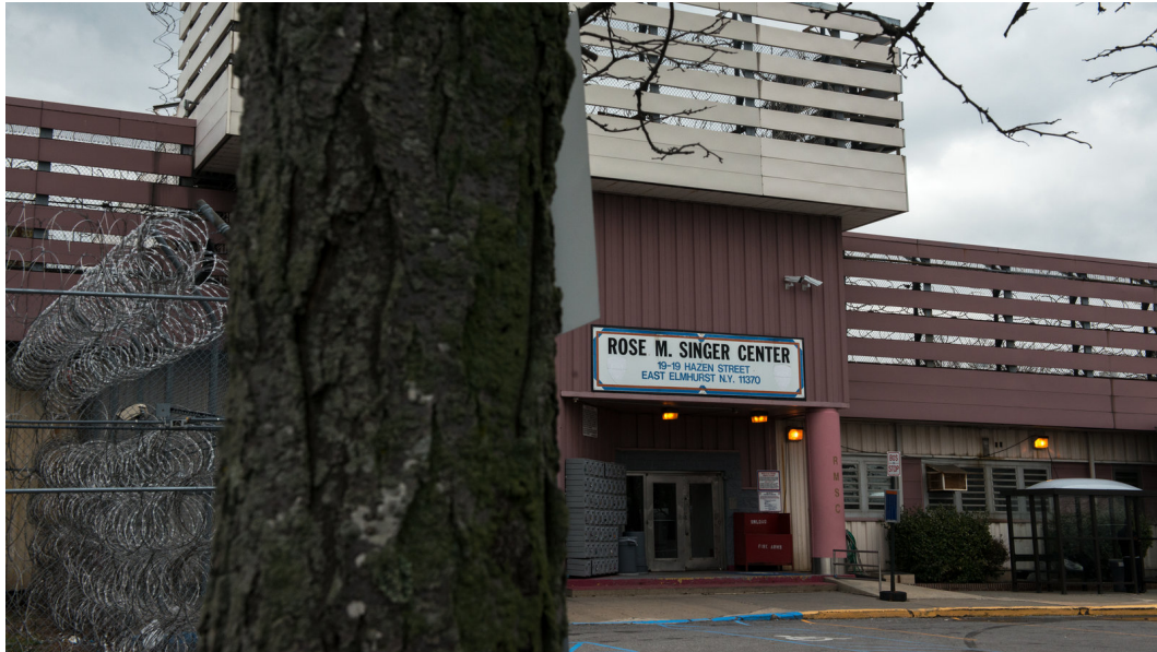
View of front entrance of RMSC
