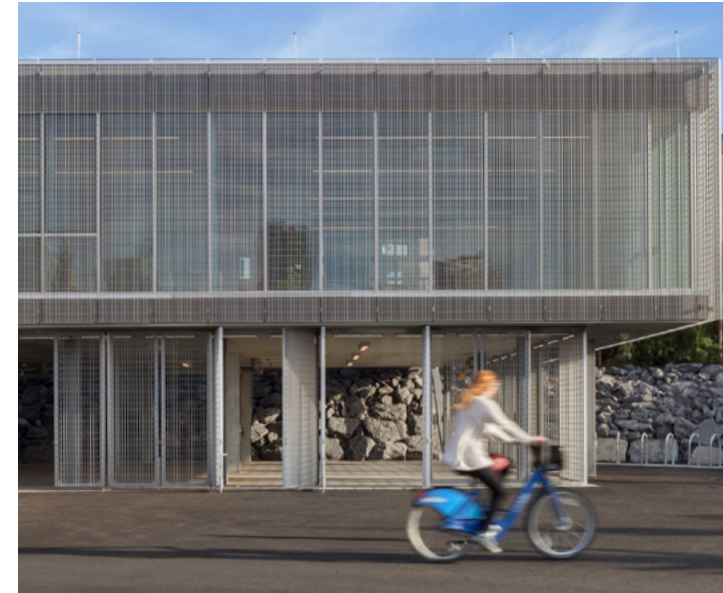
GALVANIZED METAL GRATING BROOKLYN BRIDGE BOATHOUSE
