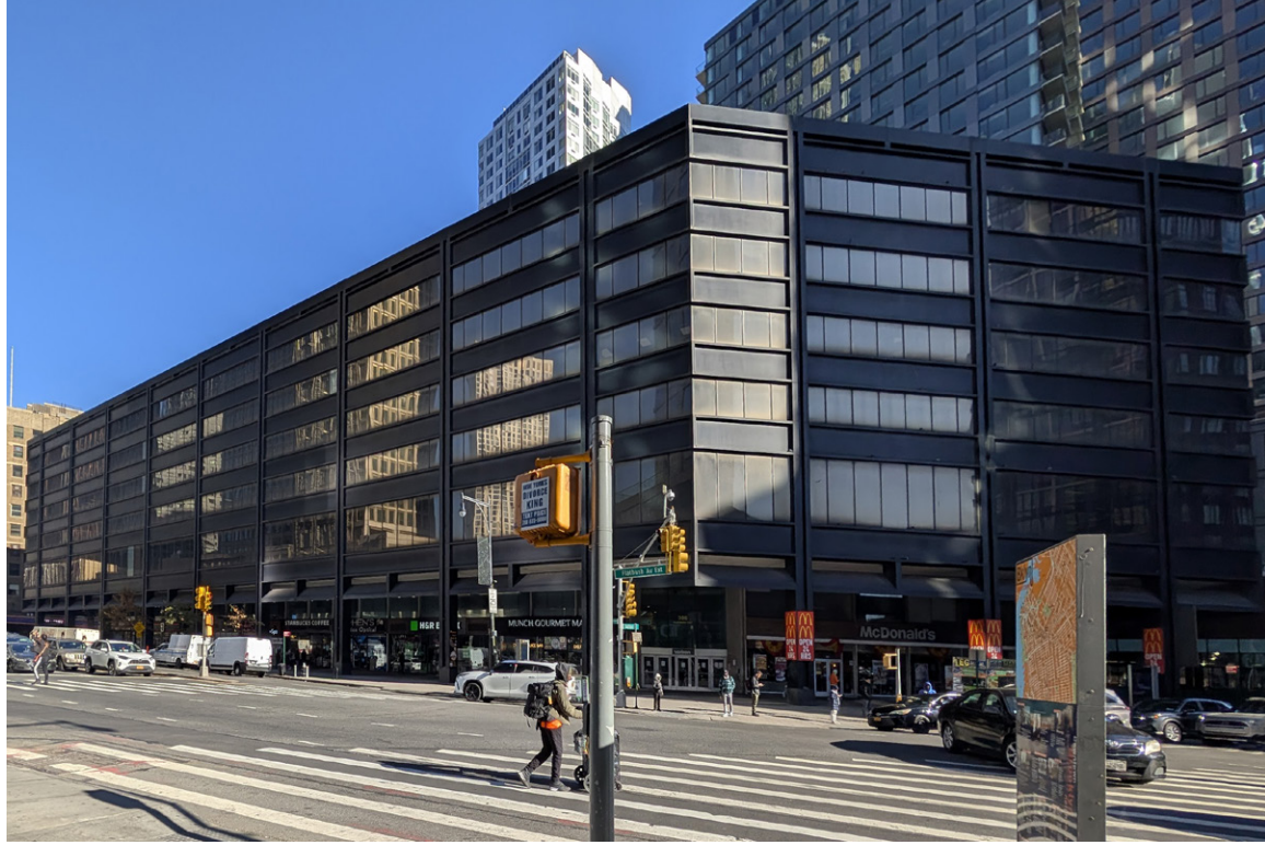
1 - NORTHEAST VIEW AT THE INTERSECTION OF FLATBUSH - FULTON
