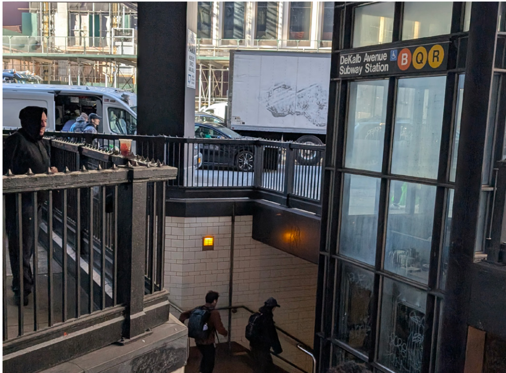
SUBWAY ENTRY OVERLOOK
