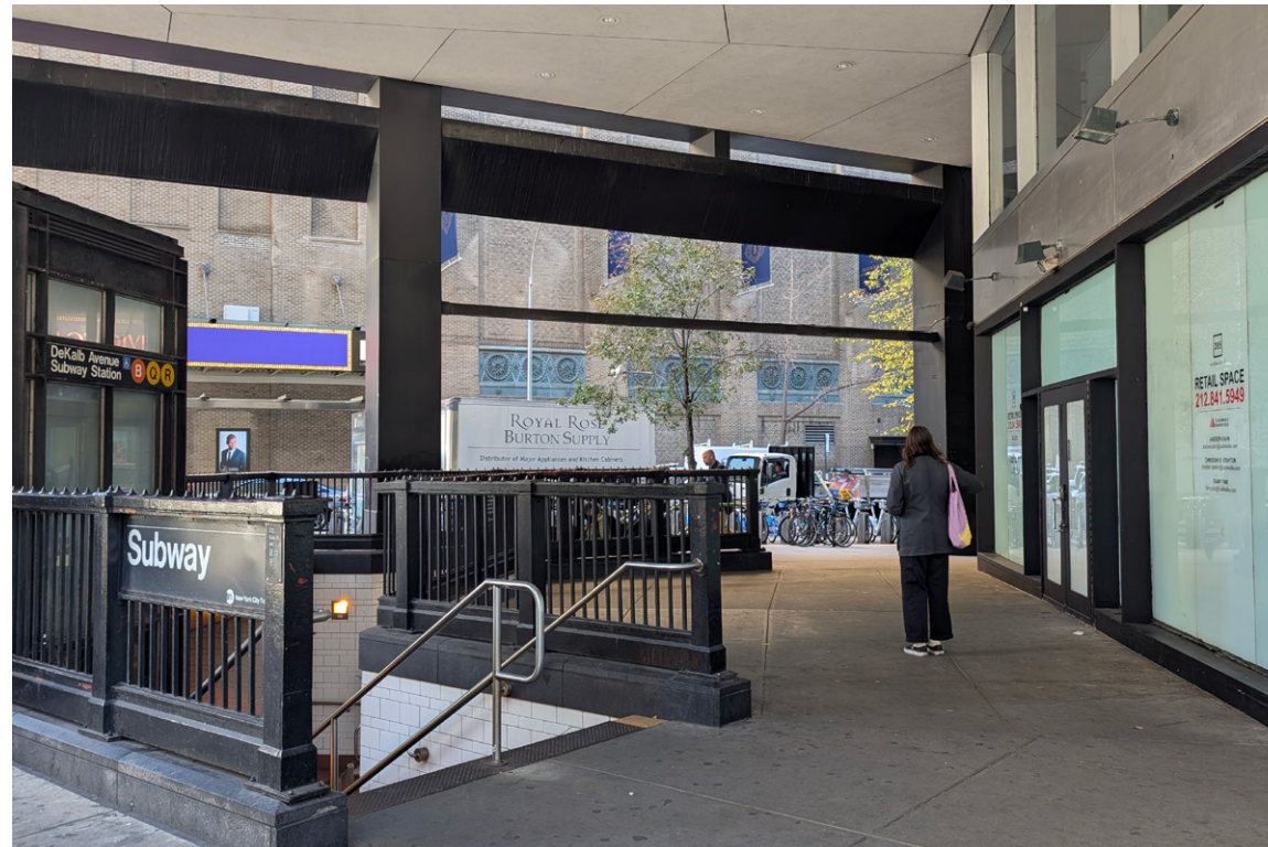
8 - EXISTING SUBWAY ENTRANCE
