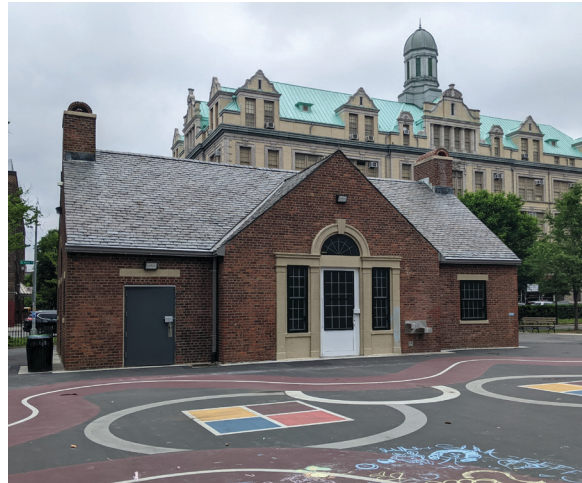
2 St. Mary's Park Comfort Station
