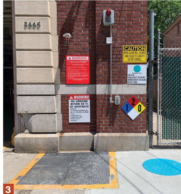
3. A standardized fuel tank access hatch and associated signage, switches, and alarms outside a Fire Department of New York Engine Company building
