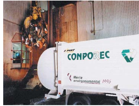
Photo 3-3: Inside the Conporec tipping building After crossing the weigh scale, trucks empty solid waste into a large waste pit.
