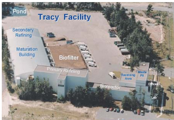
Photo 3-2: Aerial view of Conoprec Tracy MSW-composting facility Located on a nine-acre site in the Tracy Industrial Park, the actual facility footprint is approximately two acres.
