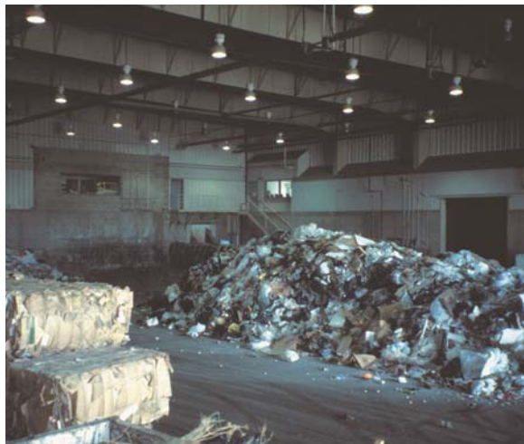
Photo 3-23: Tipping floor at the Rapid City MRF and MSW-composting facility
