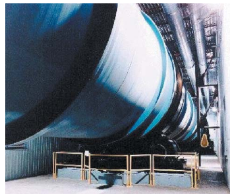
Photo 3-5: Bioreactor drum at the Conporec MSW-composting facility The drum is 14 feet in diameter, 157 feet long, and is housed entirely indoors.
