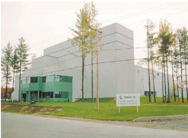
Photo 3-1: Front of the Conporec Tracy MSW-composting facility The facility is located in the City of Sorel-Tracy, 40 miles northeast of Montreal, in the Province of Quebec.
