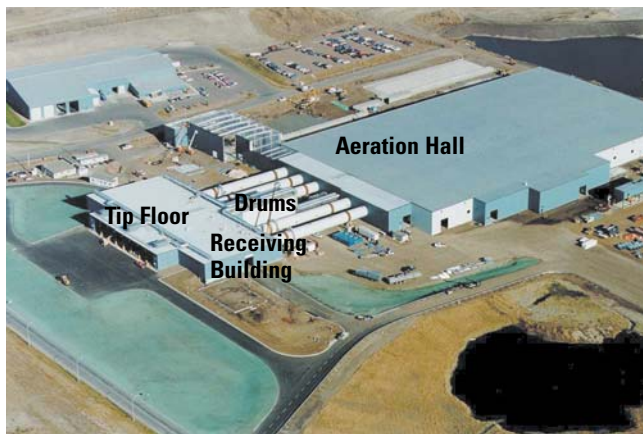
Photo 3-12: Aerial view of Edmonton facility The actual facility footprint is approximately 10 acres, which includes: receiving building, tip floor, five drums, primary screening area, aeration hall, refining area, biofilters, an office building, and parking.
