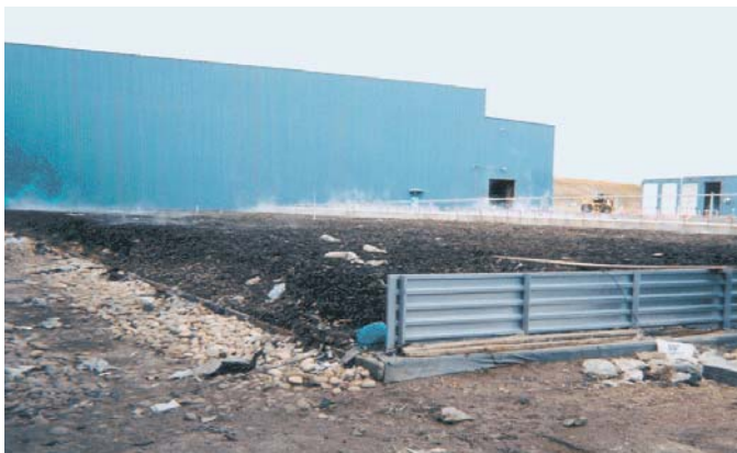
Photo 3-19: Biofilter at Edmonton facility Edmonton has three, above-ground, outdoor biofilters, which are composed of softwood bark and compost.
