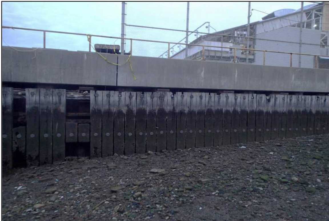
Photograph 24: East Bulkhead – Timber fender system (looking north)
