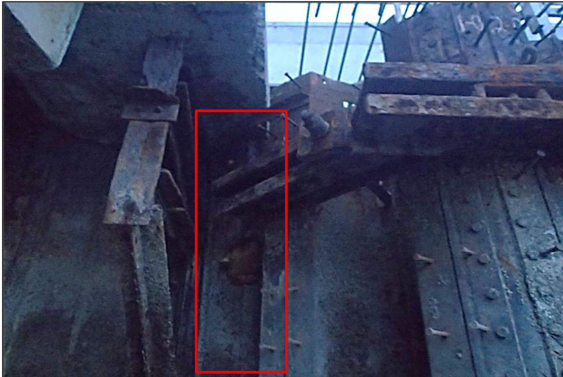
Photograph 8: North Bulkhead – Transition from steel sheet pile cell to steel sheet pile bulkhead (looking east)
