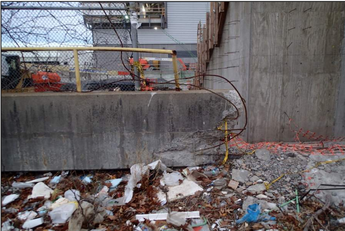
Photograph 22: East Bulkhead – Demolished concrete curb and deck at Sta. 0+14 (looking north)
