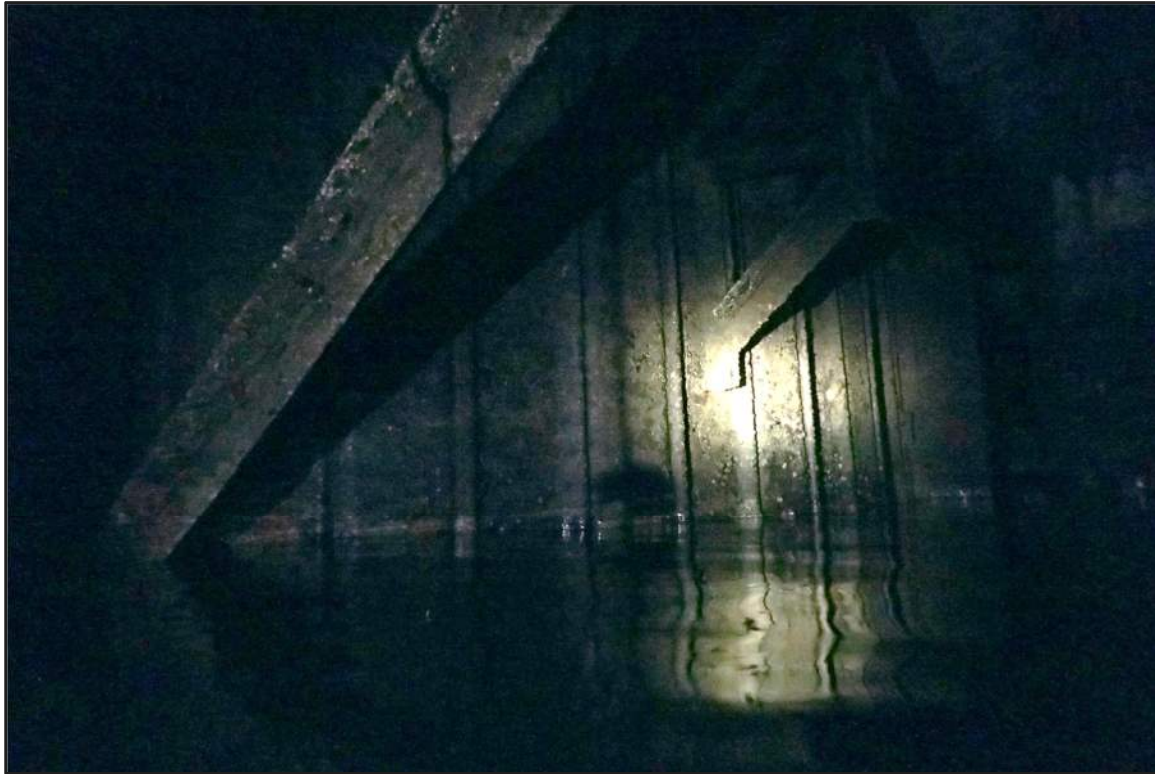
Photograph 7: North Bulkhead – Steel sheet pile cell under North Pier (looking southeast)
