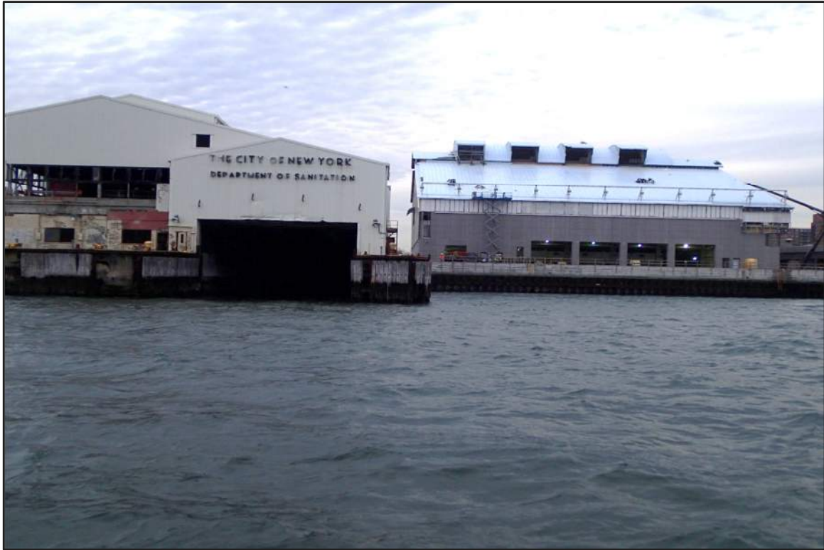
Photograph 1: Former southwest Brooklyn Marine Transfer Station and ongoing inshore construction (Looking east)
