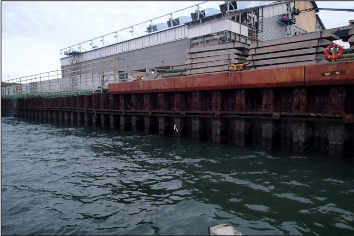
Photograph 6: Overview of the North Bulkhead (Looking northeast)
