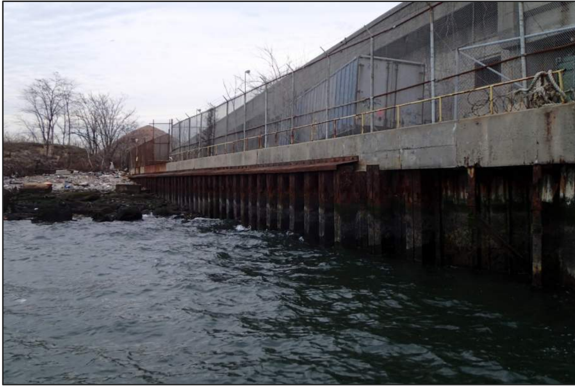
Photograph 3: Overview of the West Bulkhead (Looking southeast)
