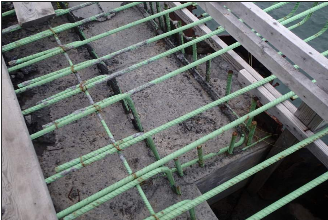
Photograph 12: North Bulkhead – Extended concrete bulkhead between Sta. 1+90 and 1+97 (Looking southwest)
