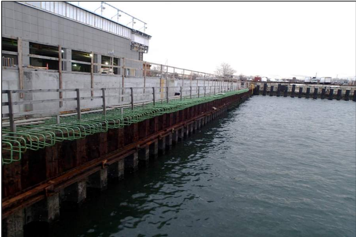
Photograph 2: Overview of the North Bulkhead and active construction site (Looking southeast)
