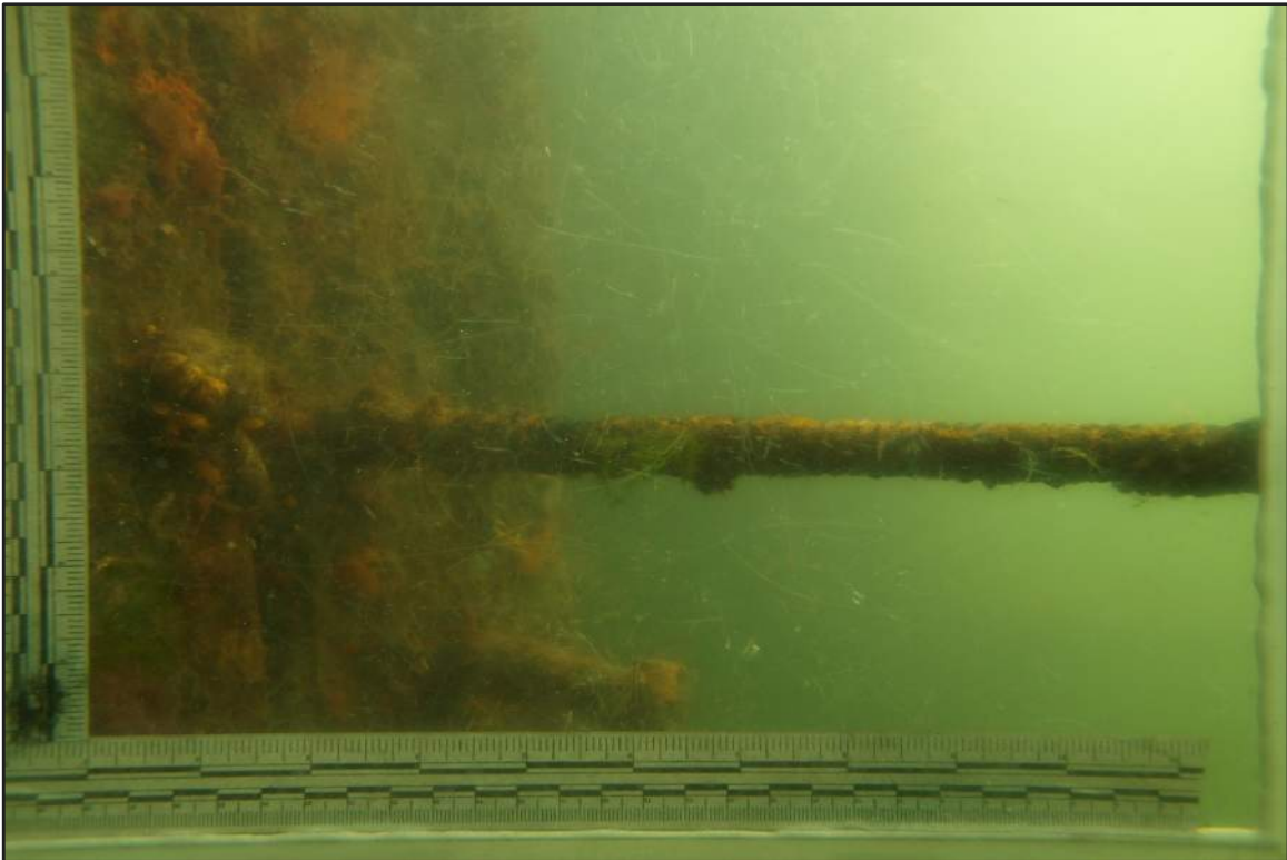
Photograph 18: North Bulkhead – Threaded rod installed between shear bolt elevations
