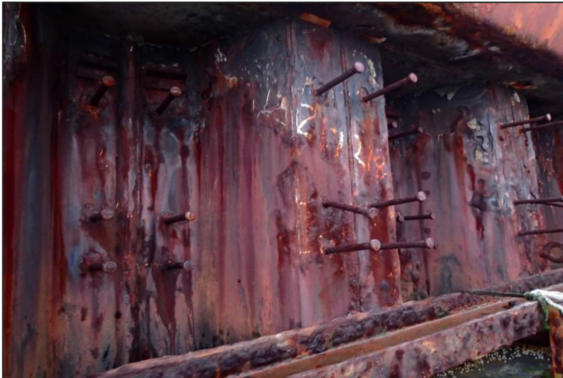
Photograph 16: North Bulkhead – Typical shear bolt installation above water (Looking southeast)
