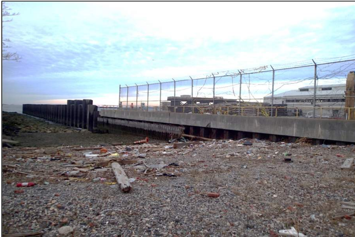
Photograph 20: Overview of the East Bulkhead (Looking northwest)
