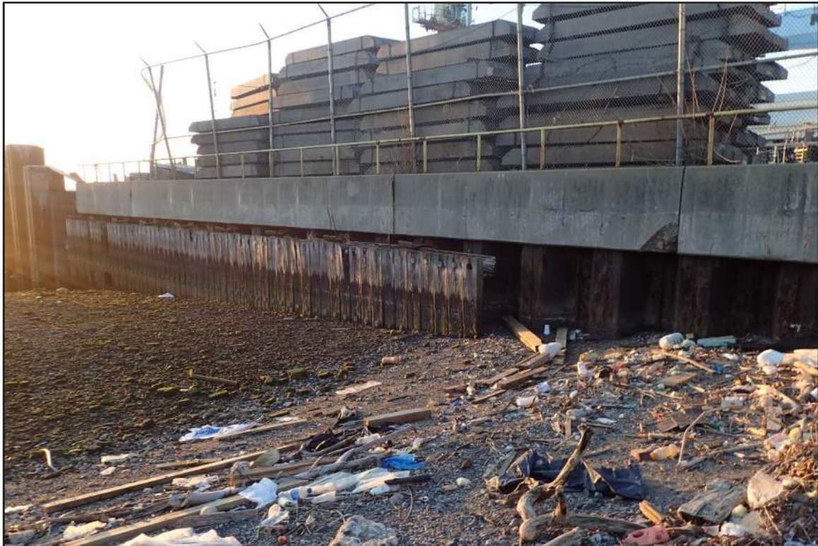
Photograph 24: Overview of the East Bulkhead (Looking northwest)
