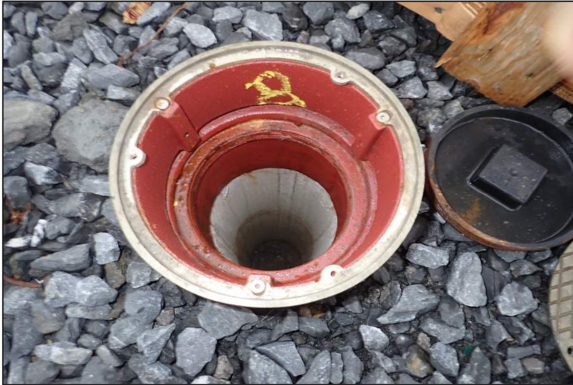
Photograph 45: North Bulkhead – Cellular cofferdam access port 8.
