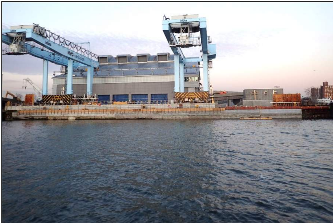
Photograph 6: Overview of the North Bulkhead (Looking northeast)
