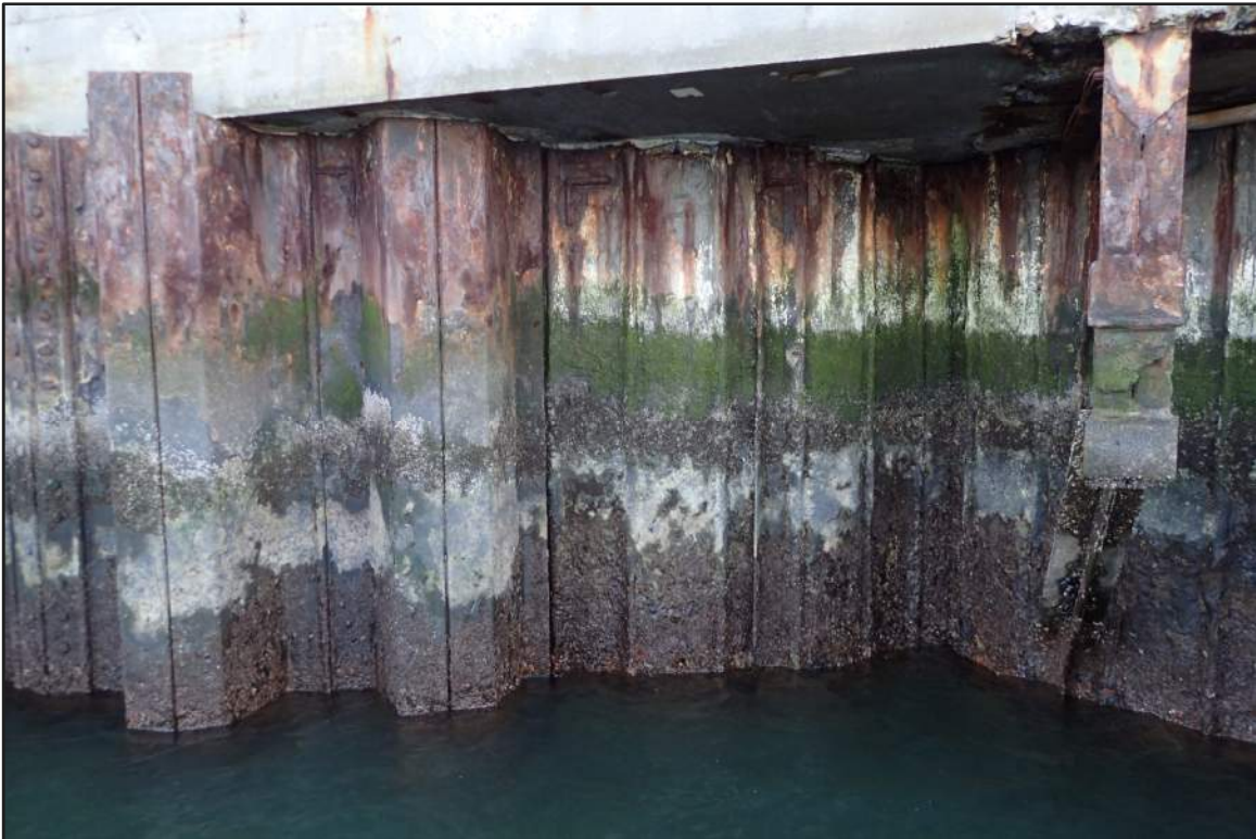
Photograph 4: West Bulkhead - Steel sheet pile cell interface with steel sheet pile bulkhead (Looking southeast)
