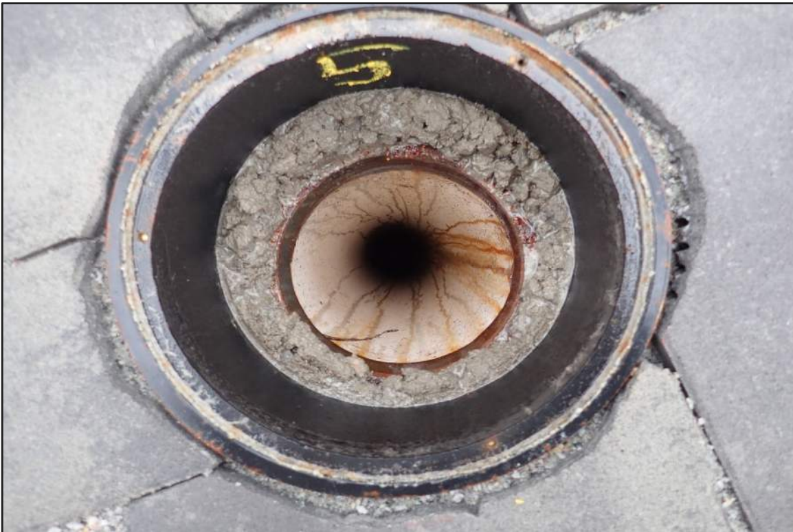
Photograph 44: North Bulkhead – Cellular cofferdam access port 5.
