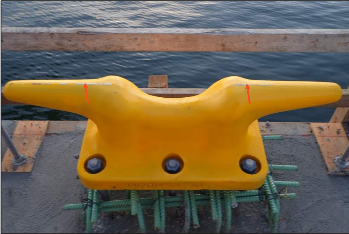
Photograph 43: North Bulkhead - Typical minor coating loss of new mooring hardware cleat due to abrasion during installation process (Looking west)
