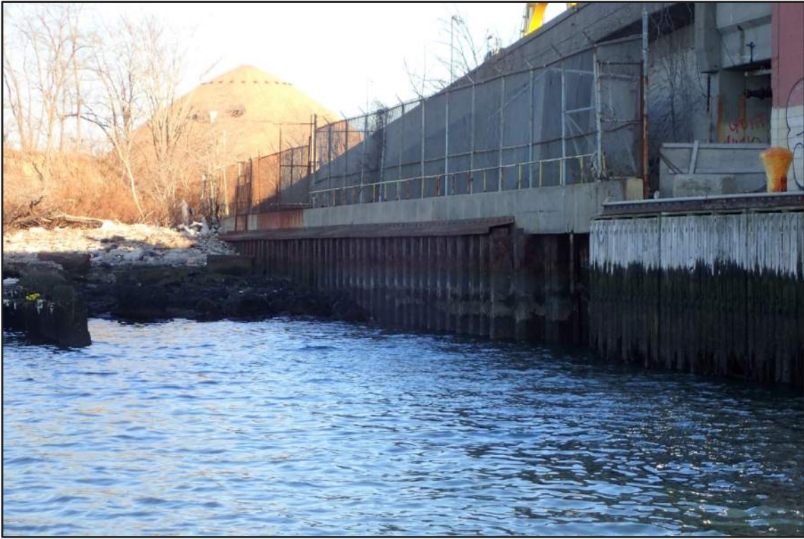
Photograph 3: Overview of the West Bulkhead (Looking east)
