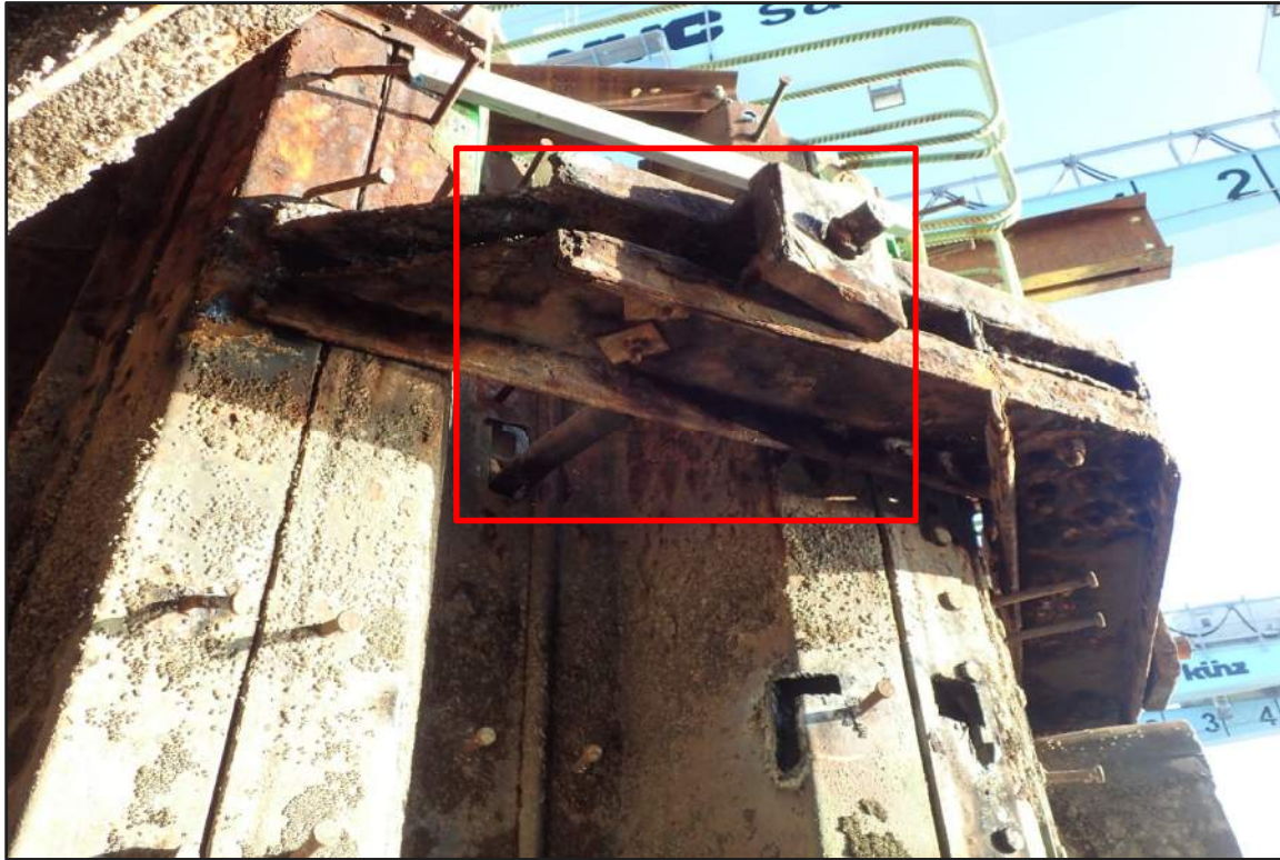
Photograph 9: North Bulkhead - Typical steel double channel wale, anchor rod, and hardware (Looking southeast)
