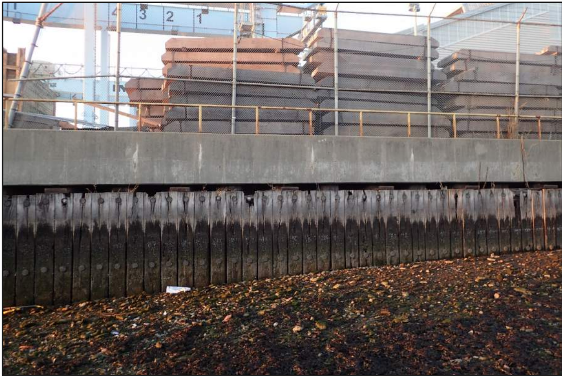
Photograph 27: East Bulkhead – Timber fender system (Looking north)
