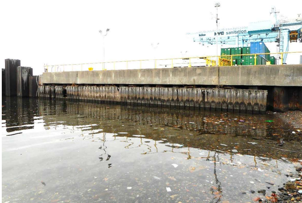
Photo 2-9. Western Bulkhead and Fender at New SW Brooklyn MTS
