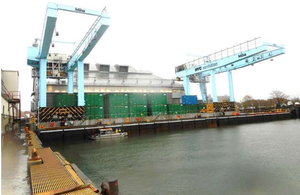
Photo 2-2. New SW Brooklyn MTS (Looking East)
