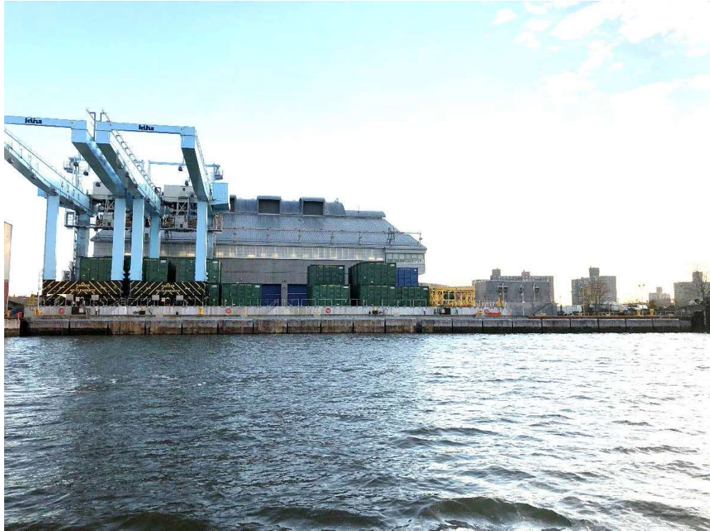
Photo 2-7. New SW Brooklyn MTS (Looking East)
