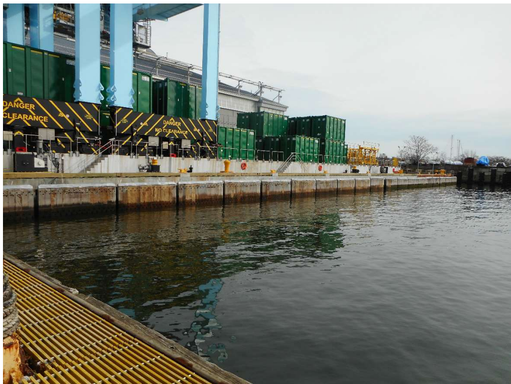
Photo 2-8. Western Bulkhead and Fender at New SW Brooklyn MTS
