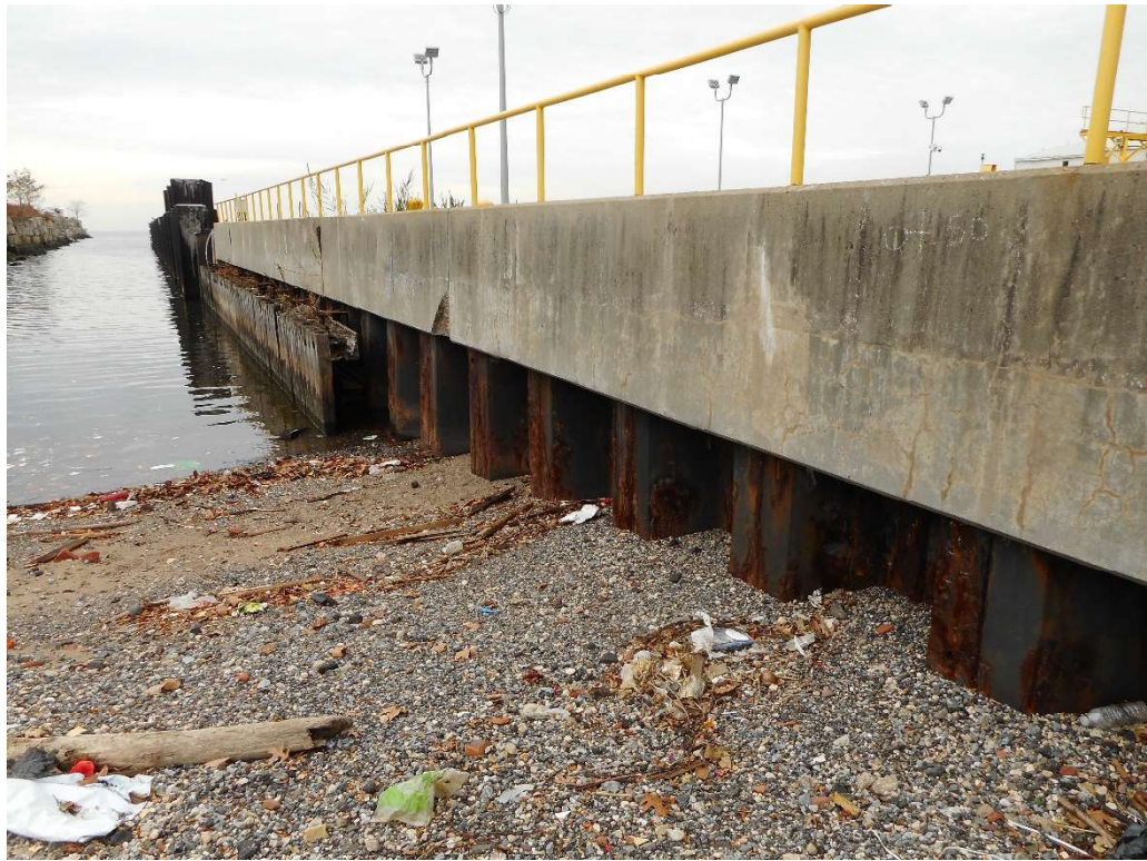
Photo 3-110. South Face of Western Bulkhead
