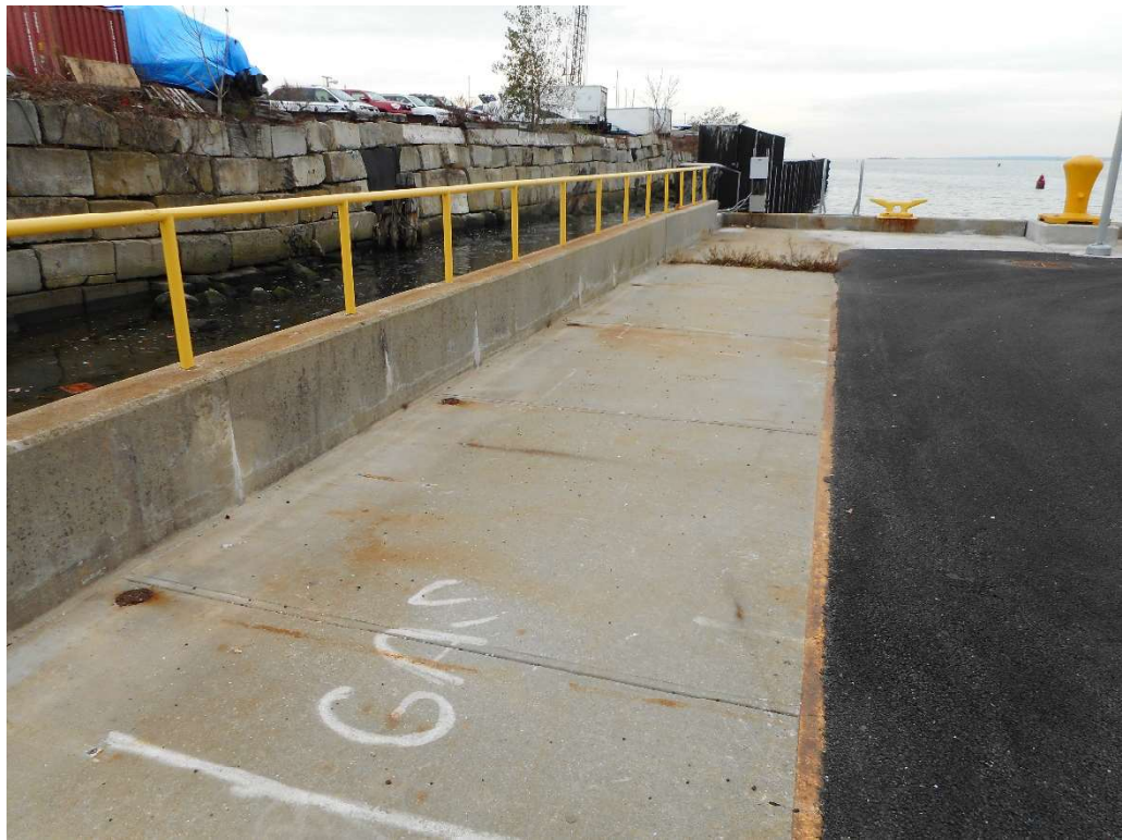
Photo 3-111. Pile Cap and Concrete Deck at Western Bulkhead (South Face)
