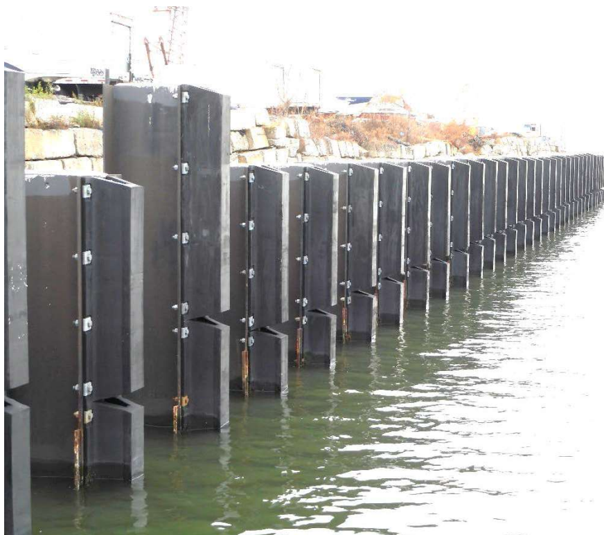
Photo 2-10. Southwest Bulkhead and Fender at New SW Brooklyn MTS
