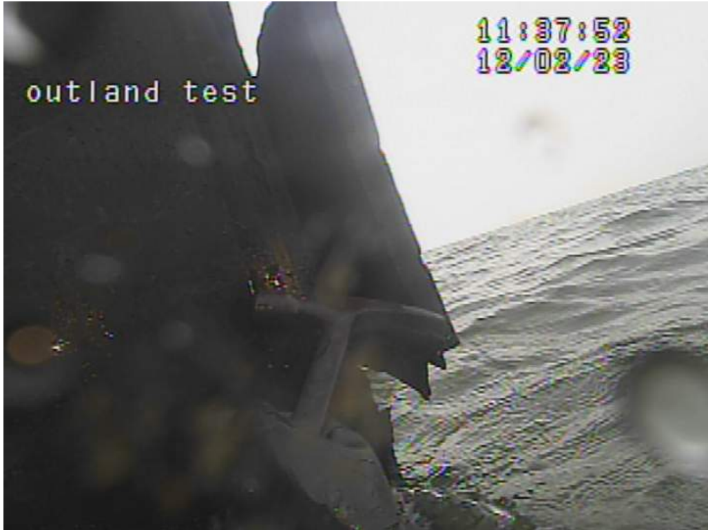
Photo 5. Rubber Fender Peeling Off.
