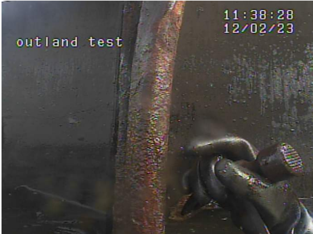
Photo 6. Bent at Steel Sheeting.
