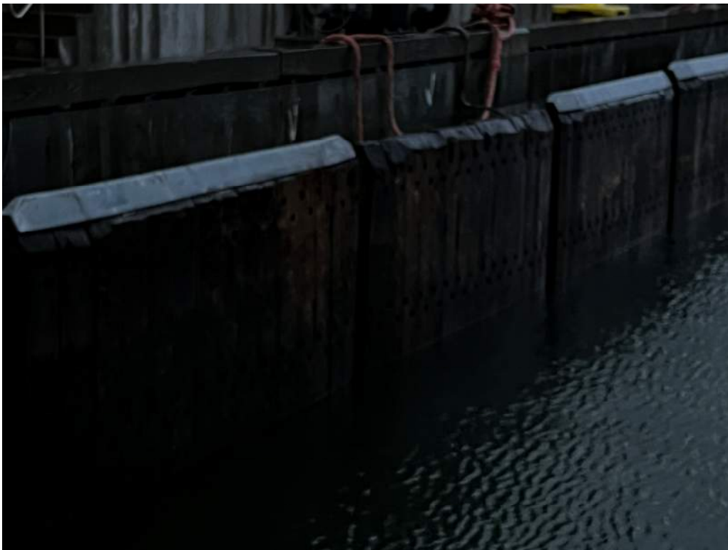
Photo 2. HDG cap plate missing at fender #3
