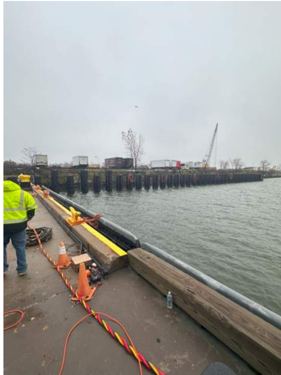
Photo 1. Overall view of East Bulkhead
