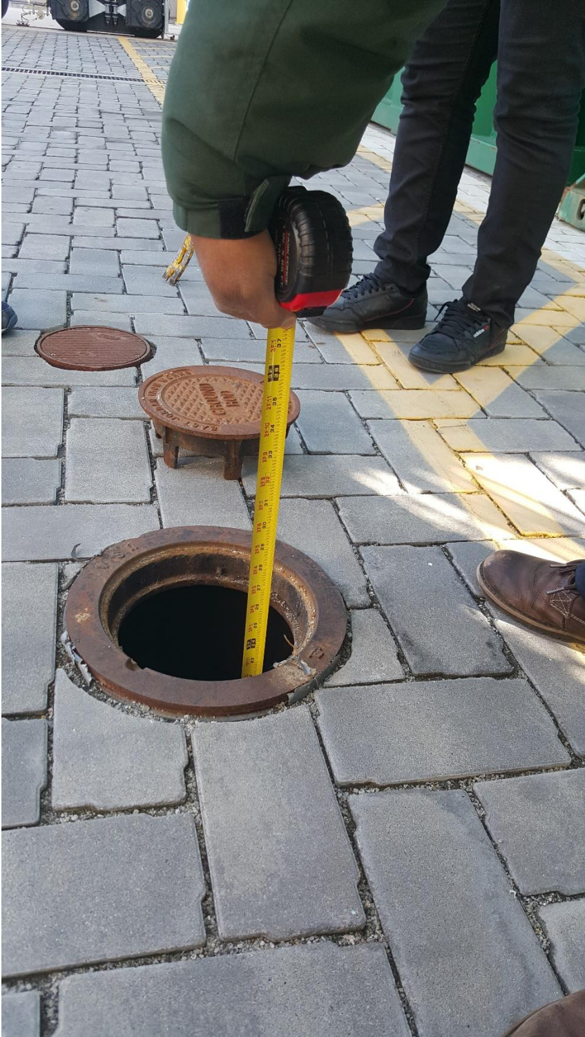
Photo 4 – Inspection Port on Pier Deck
