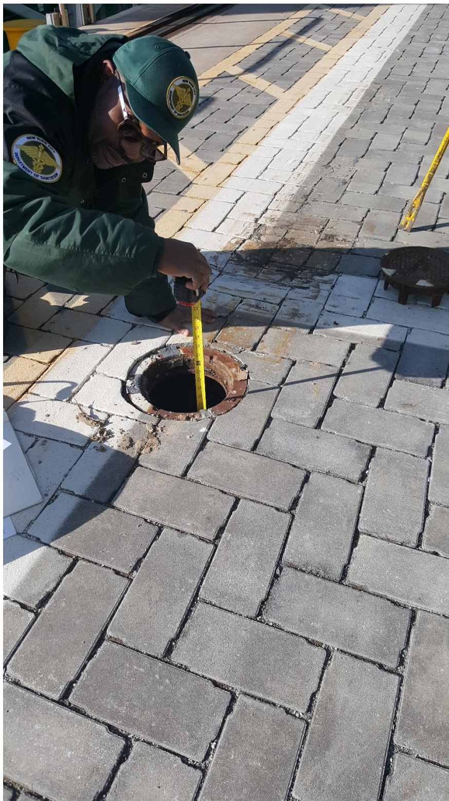
Photo 2 – Measurement Tape Lowered into Inspection Port
