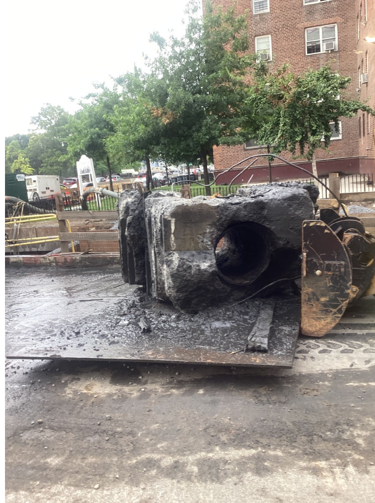
Removal of existing sewer interceptor – July 2024
