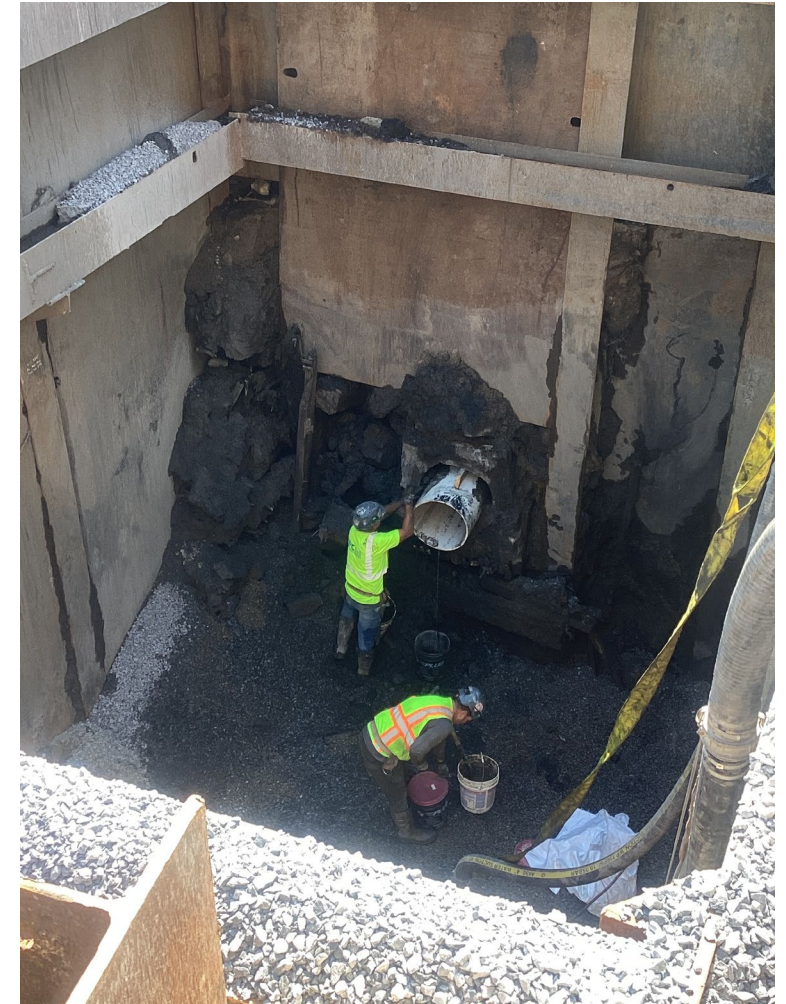
Excavation trench for microtunneling – July 2024
