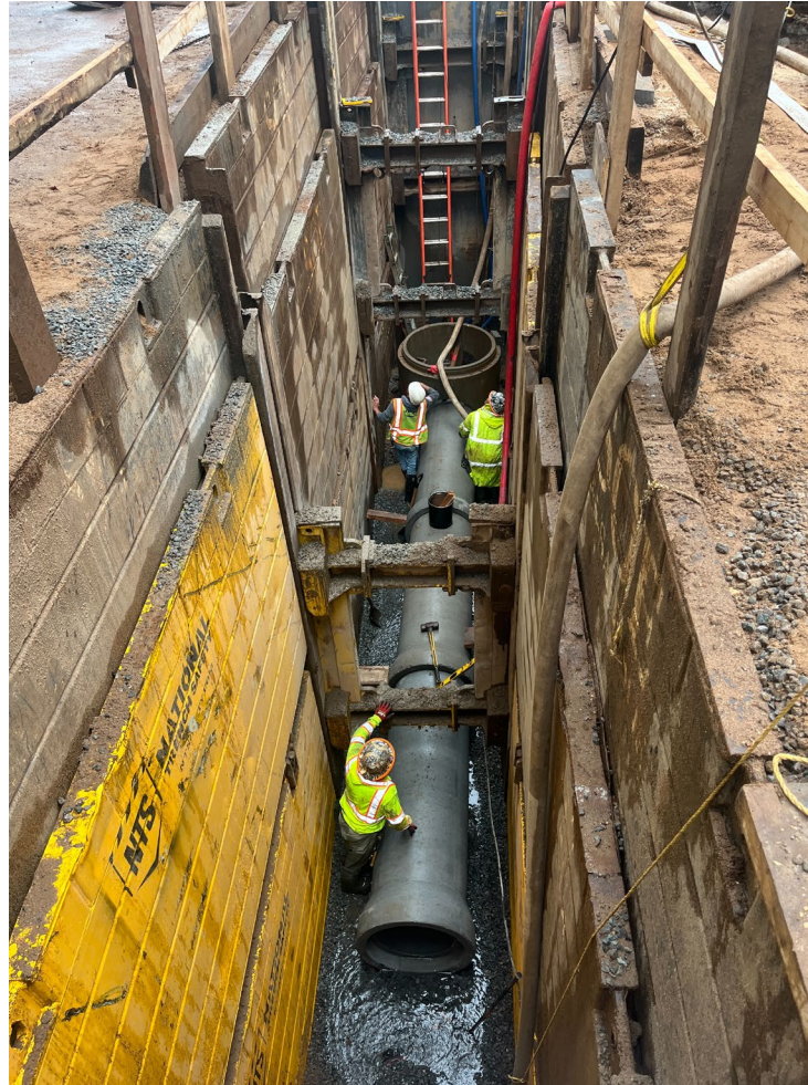
Sewer installation on Water Street – August 2024
