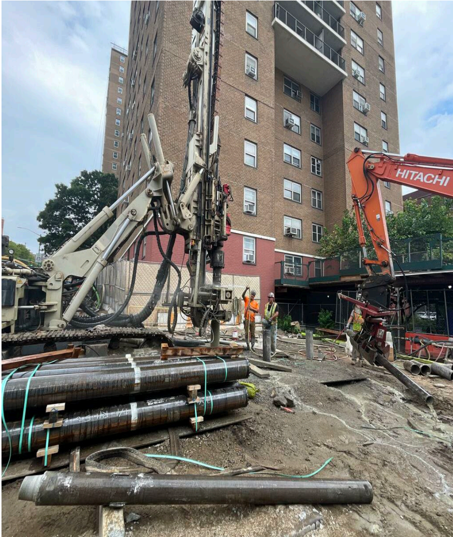
Pressure grouting soil at Gouverneurs Garden
