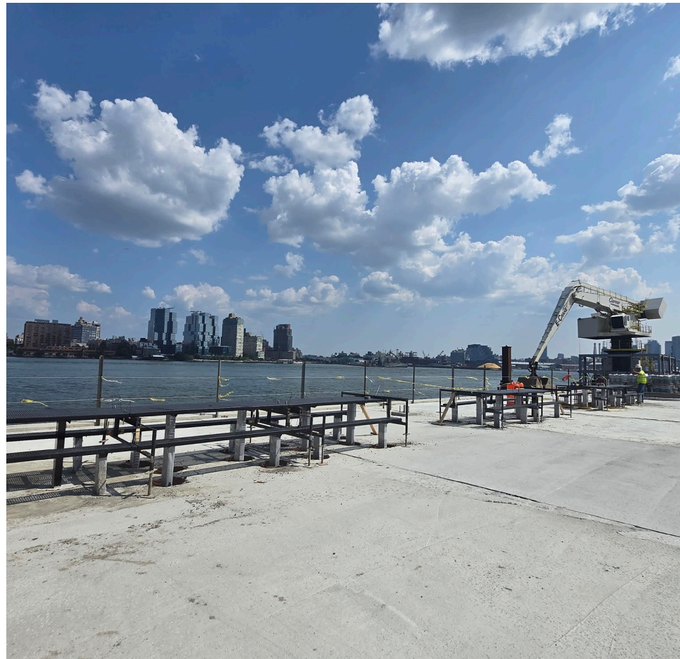
Benches and tables being installed near BBQ Area – August 2024
