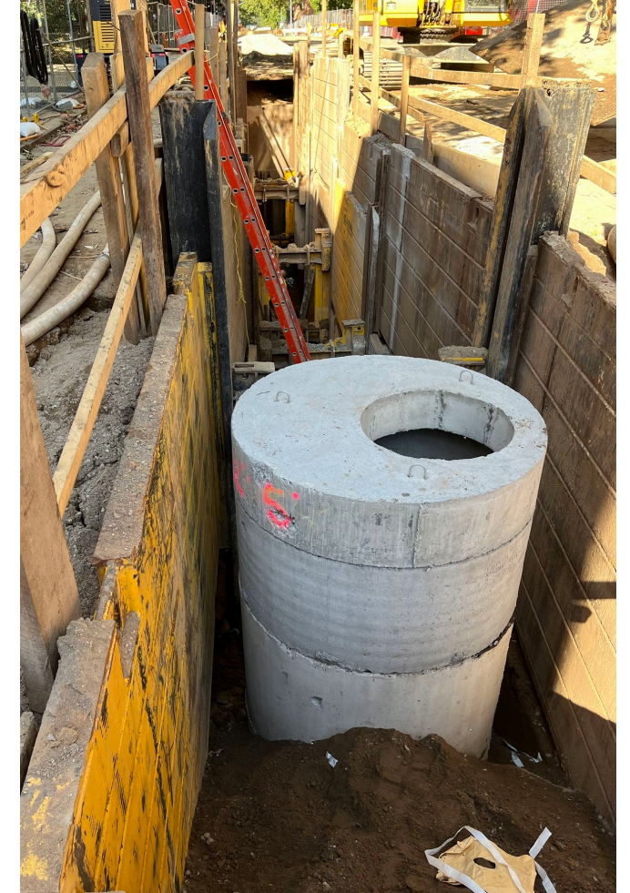
Manhole installation on Water Street – August 2024
