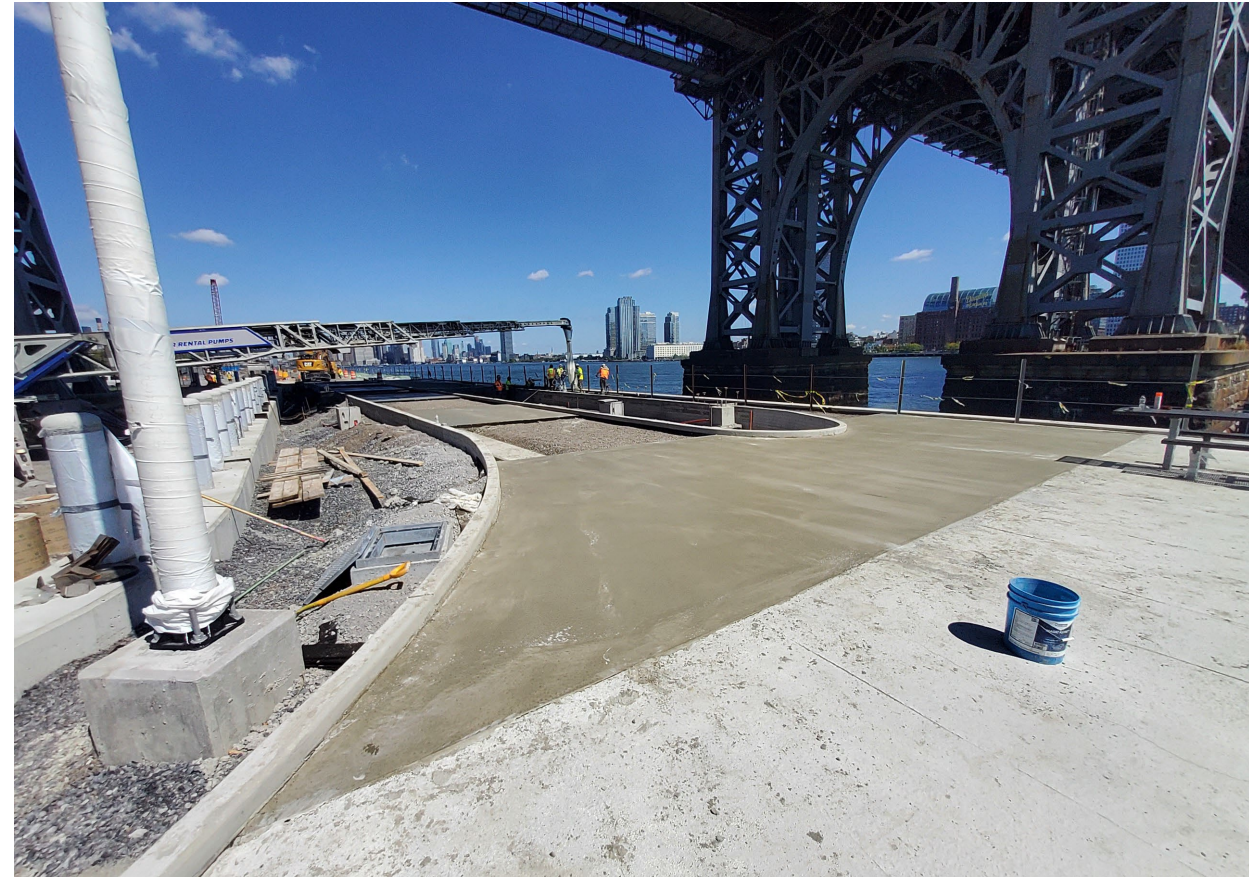
Concrete poured in esplanade area under Williamsburg Bridge – September 2024
