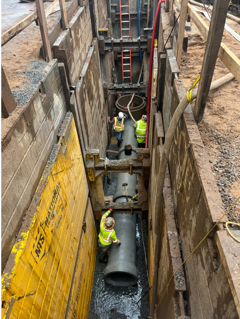
Sewer installation on Water Street – August 2024
