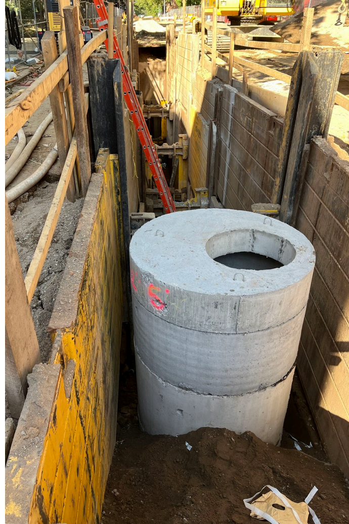
Manhole installation on Water Street – August 2024
