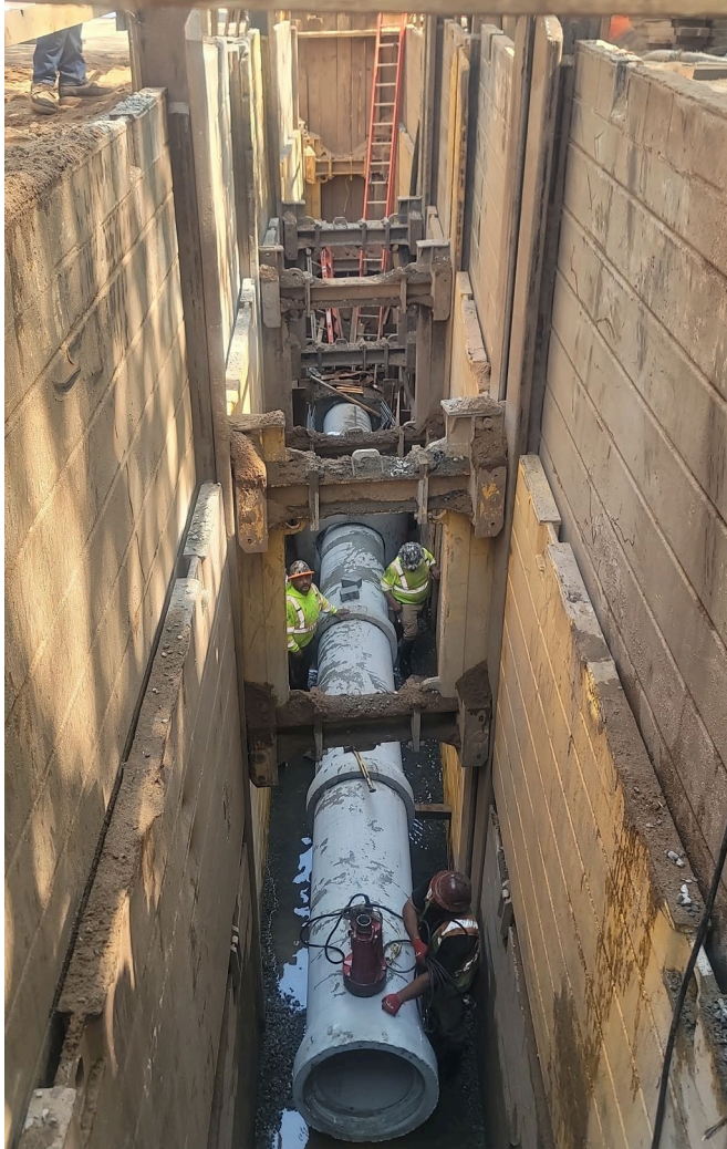
Sewer installation on Water Street – September 2024
