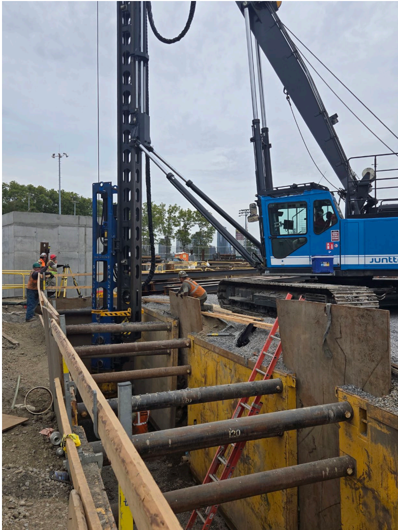
Pile driving at Ballfields 3, 4, 5 – September 2024
