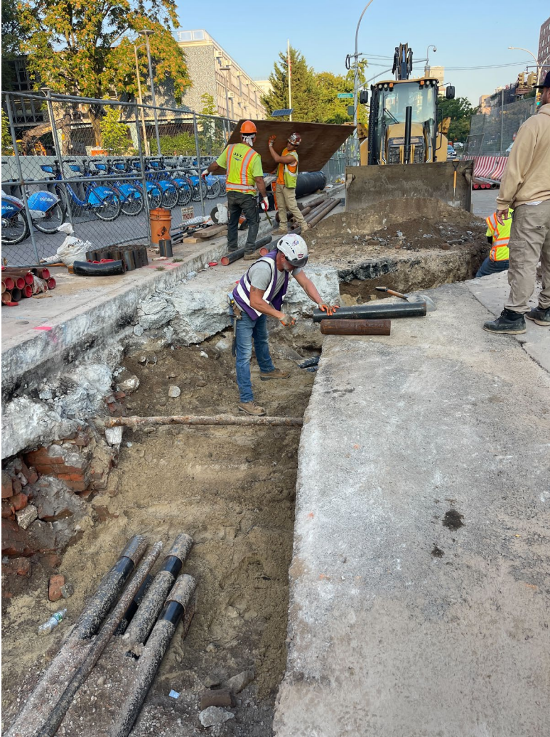
Excavation for conduit installation at E Houston St. & Columbia St. - September 2024
