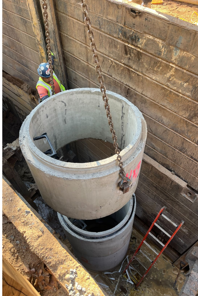
Manhole installation on Water Street – September 2024
