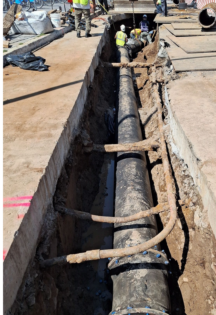
Water main installation at E Houston St. & Columbia St. - September 2024
