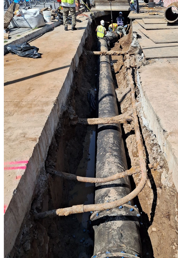
Water main installation at E Houston St. & Columbia St. – September 2024
