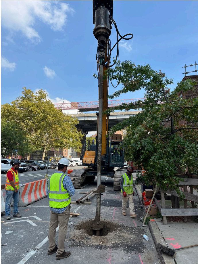
Installation of test piles on Delancey Street South -- September 2024
