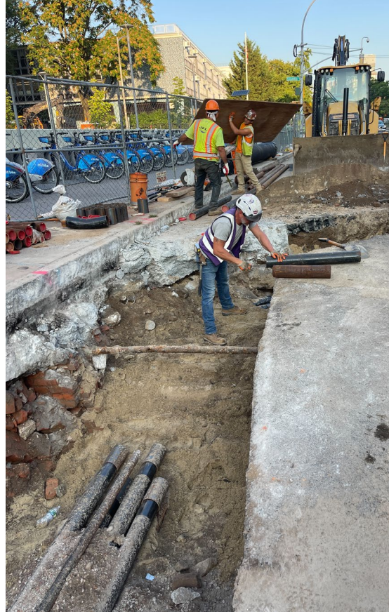
Excavation for conduit installation at E Houston St. & Columbia St. – September 2024
