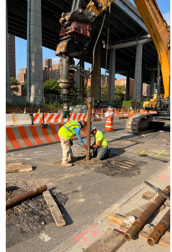
Helical pile installation on Delancey St. N – September 2024
