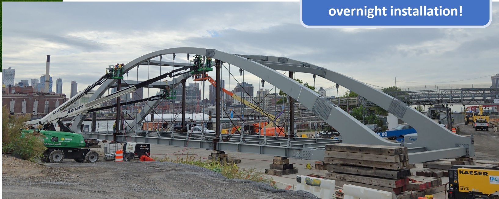
Corlears Hook Pedestrian Bridge assembly – September 2024
