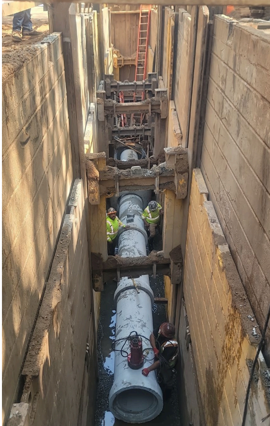
Sewer installation on Water Street – September 2024
