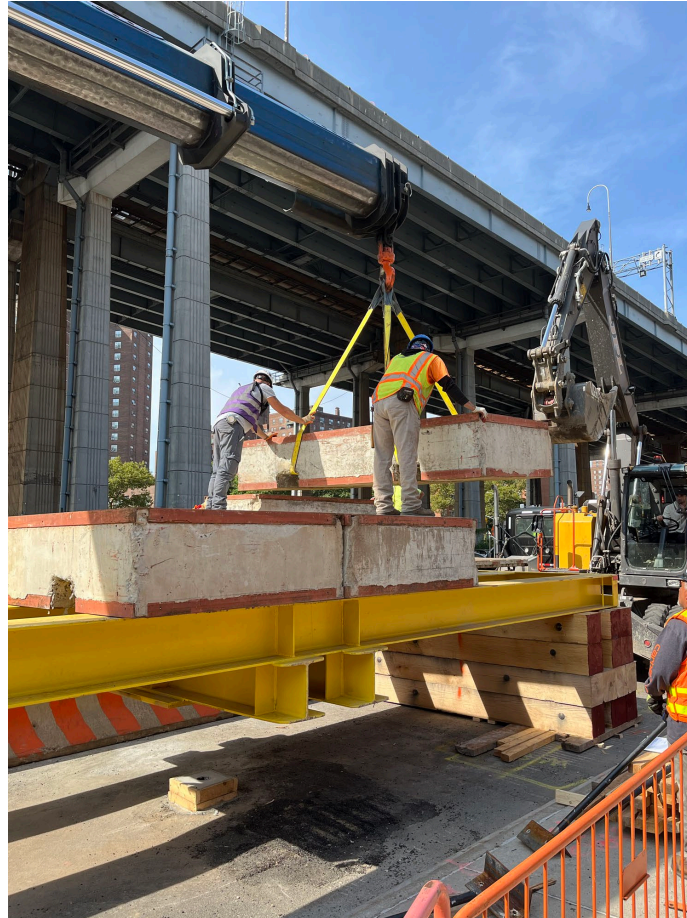
Load testing on Delancey Street South -- September 2024
