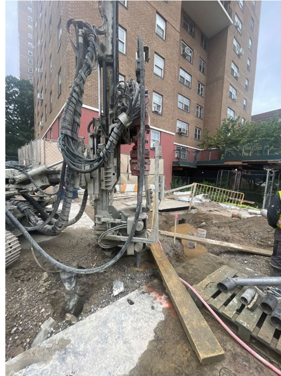
Jet grouting for future roller floodgate, September 2024
