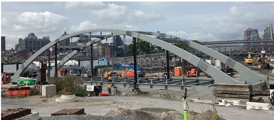
Corlears Hook Pedestrian Bridge assembly in East River Park, Sept. 2024
