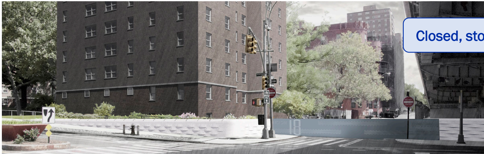
Rendering of floodwall and roller floodgate at Montgomery St. and South St.
