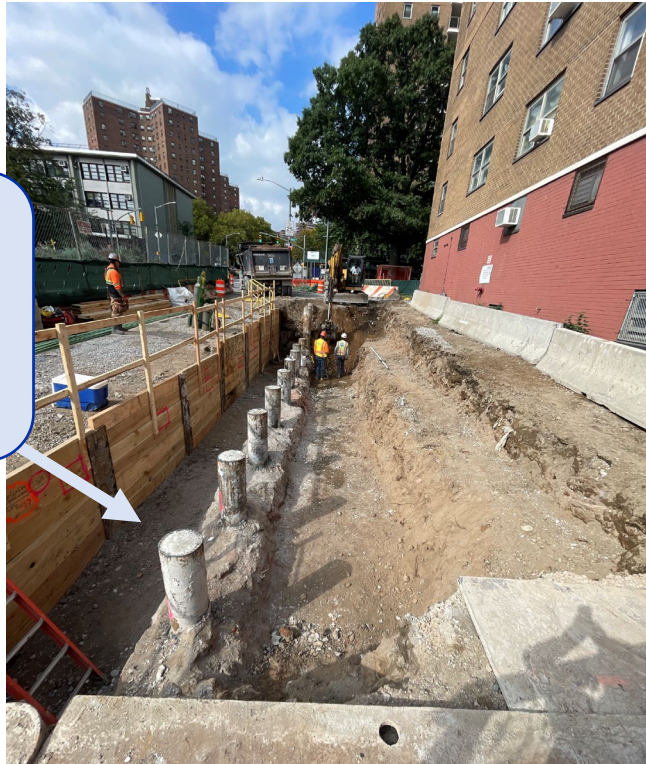
Excavation for floodwall, October 2024
