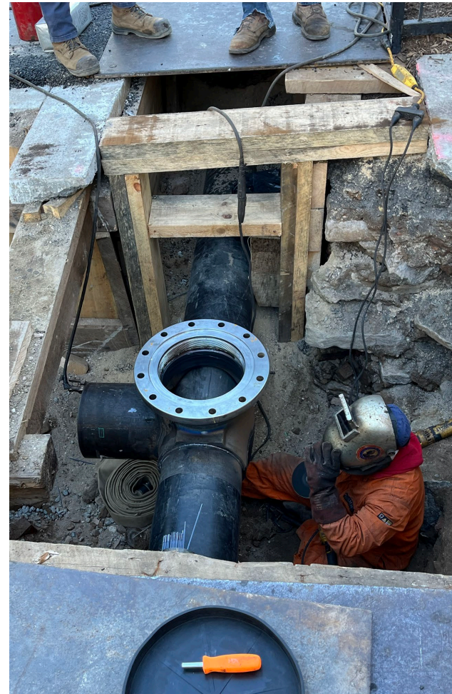
Gas main installation at Columbia St. and E. Houston St. – October 2024
