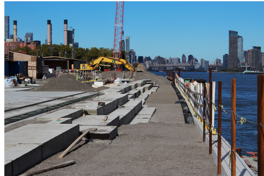
Esplanade seating foundation installation – October 2024
