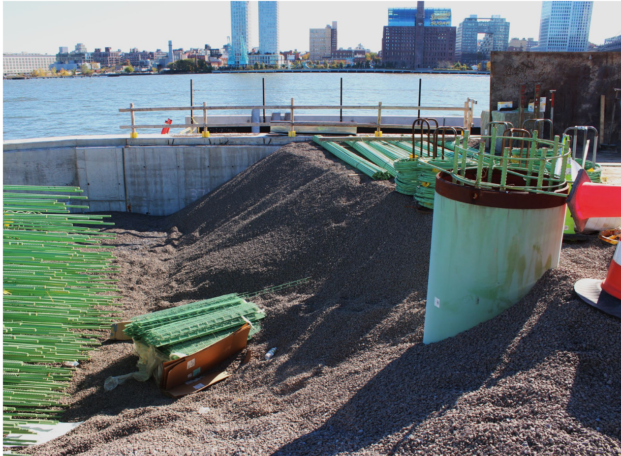
Partial fill at Esplanade near Tennis Area – October 2024
