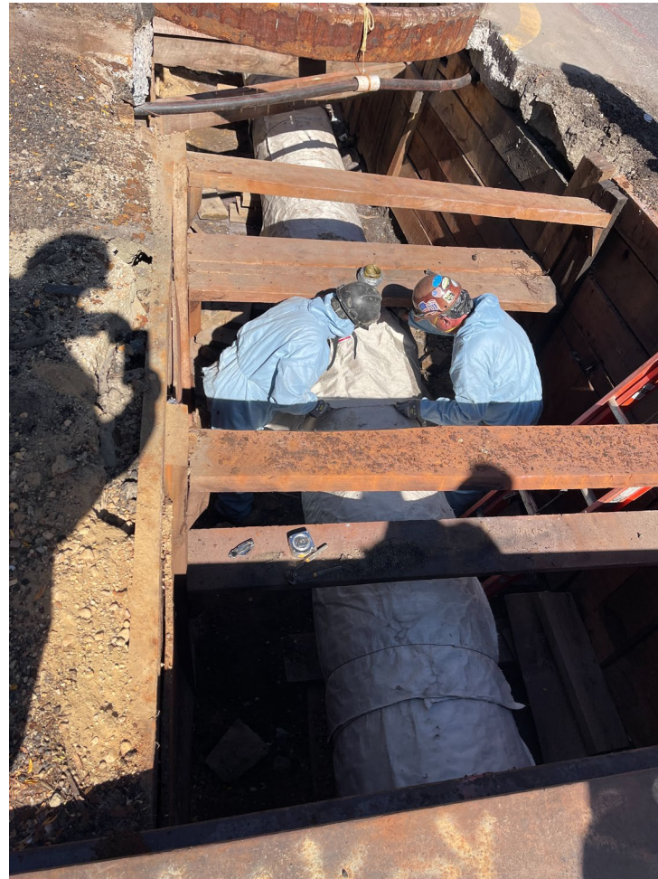
Steam main installation at E. 18 th St. and Ave C – October 2024
