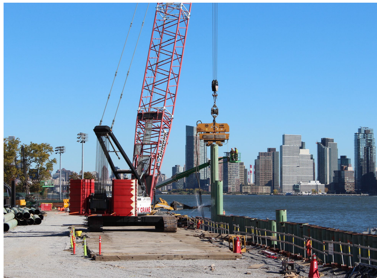
Pipe pile driving near Ballfield 5 – October 2024
