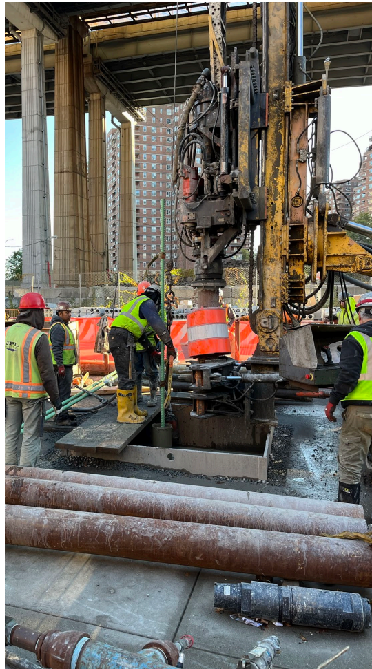
Test pile on Delancey St. N – October 2024
