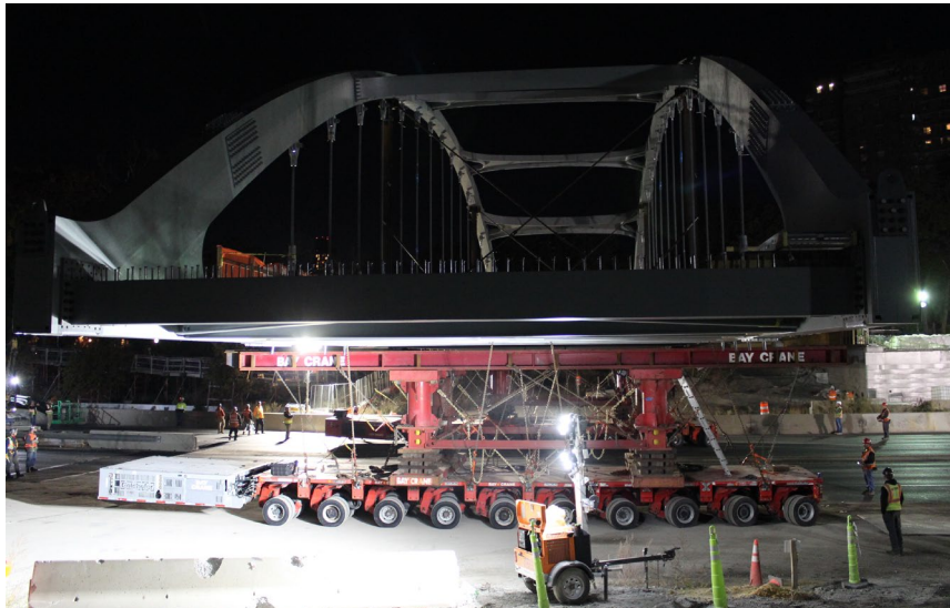
Corlears Hook Bridge rolled via SPMTs along FDR Drive during overnight closure – October 2024
