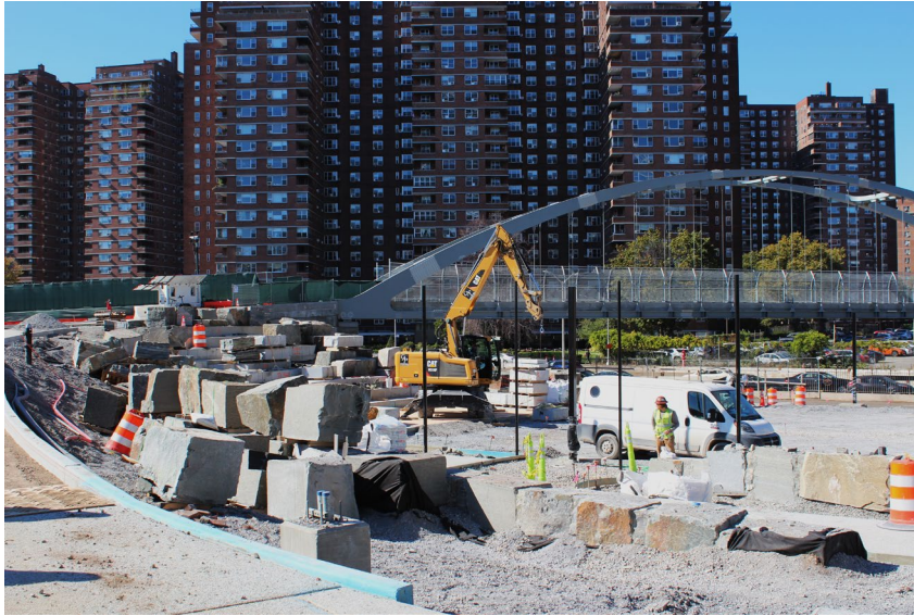
Basketball Court construction – October 2024
