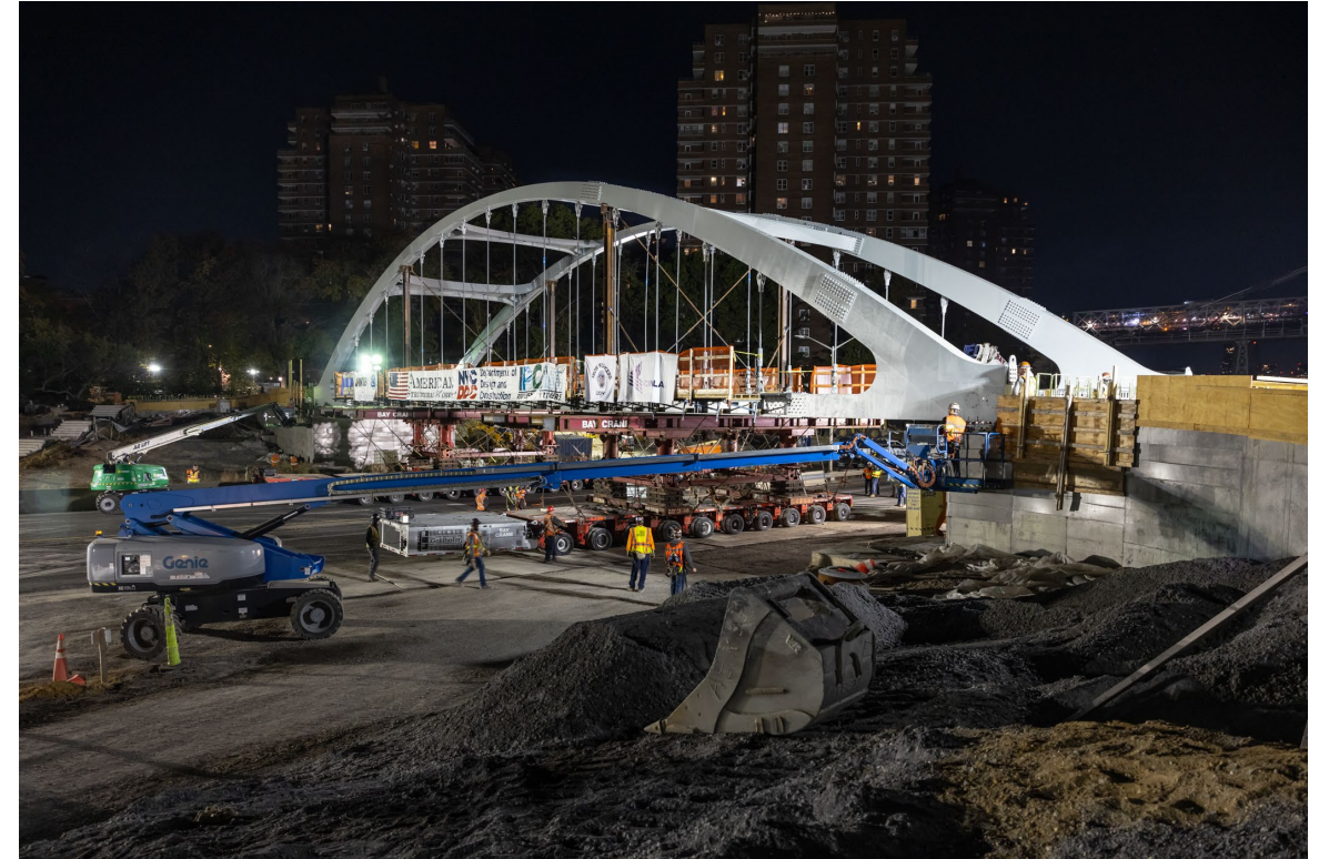
Corlears Hook Bridge being installed on abutments – October 2024
