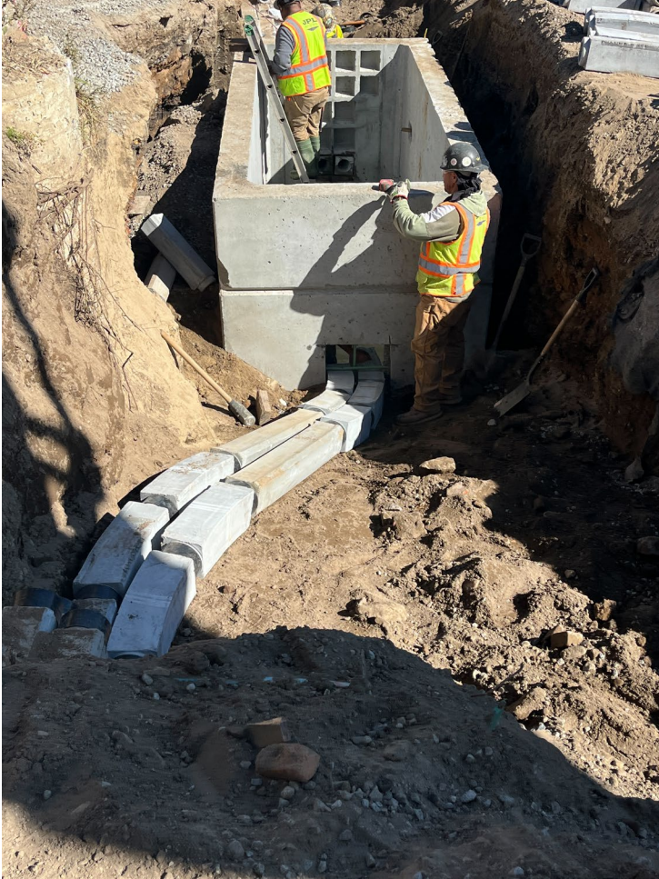
Con Ed manhole and duct installation near Corlears Hook Park – October 2024
