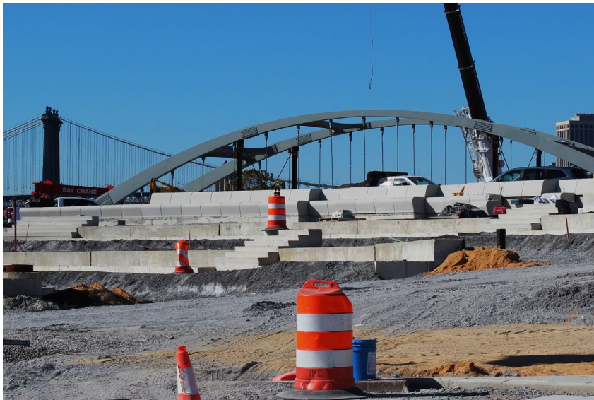
Amphitheater seating installation – October 2024
