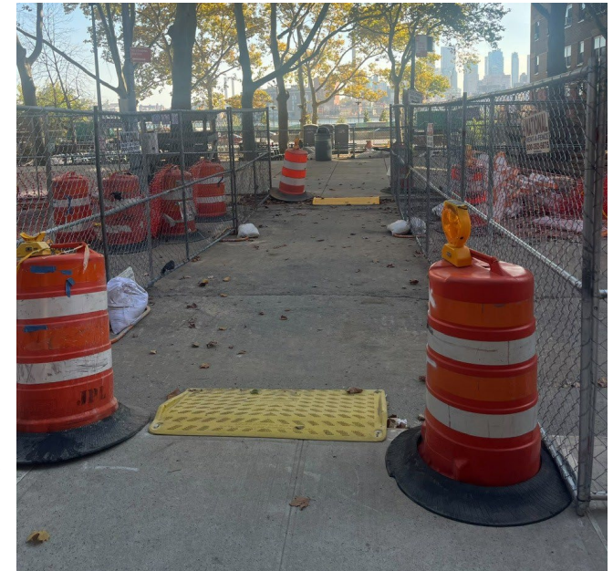
Temporary Water St. sidewalk detour (looking south) – October 2024
