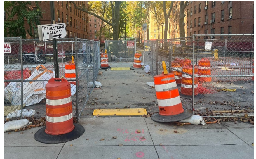
Temporary Water St. sidewalk detour (looking north) – October 2024
