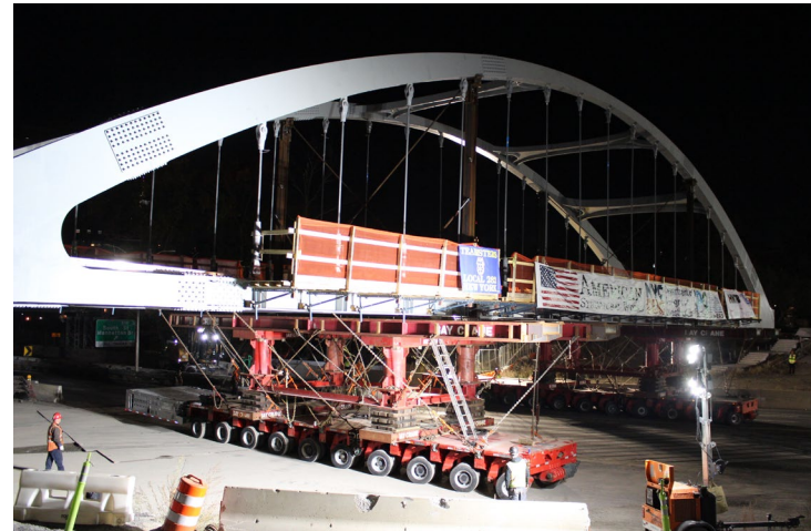
Corlears Hook Bridge rolled via SPMTs along FDR Drive during overnight closure – October 2024
