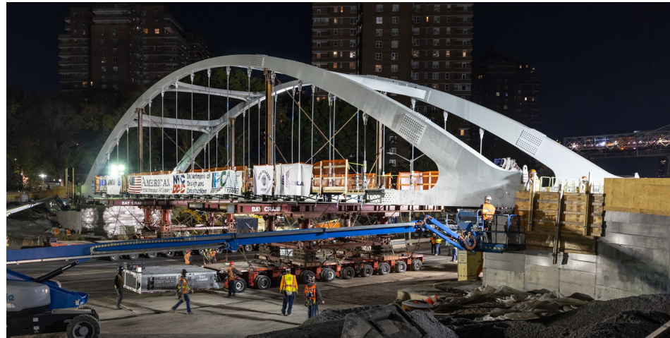
Corlears Hook Bridge being installed on abutments – October 2024
