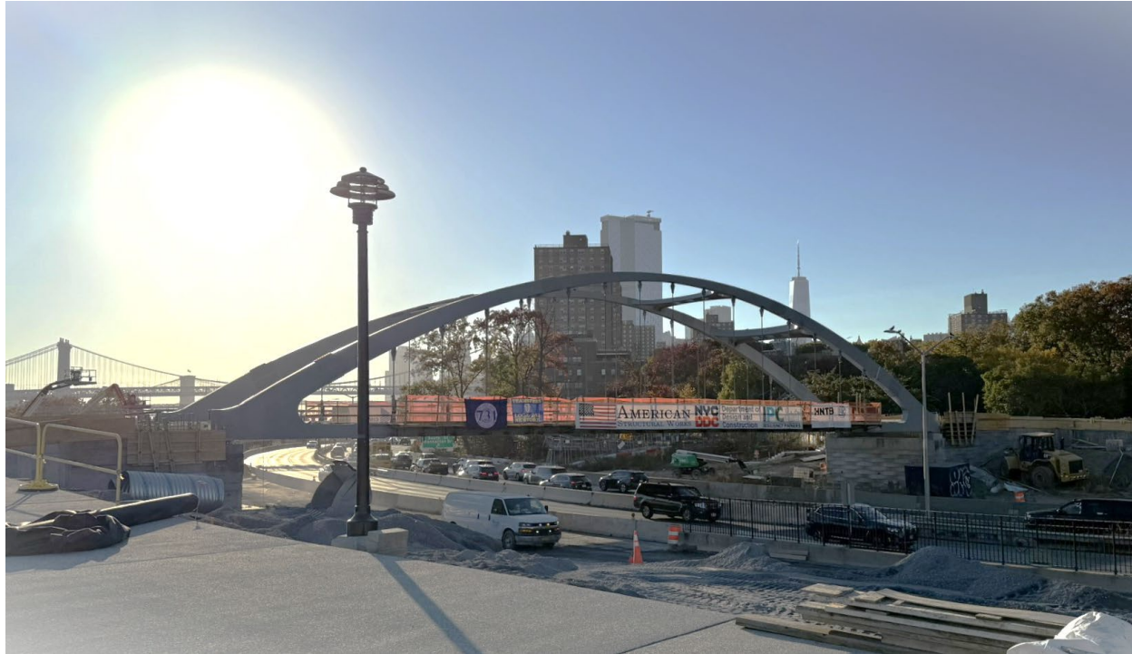
Corlears Hook Bridge after installation – October 2024
