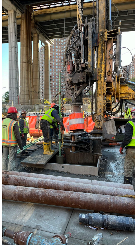
Test pile on Delancey St. N – October 2024
