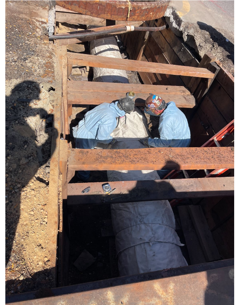
Steam main installation at E. 18 th St. and Ave C – October 2024
