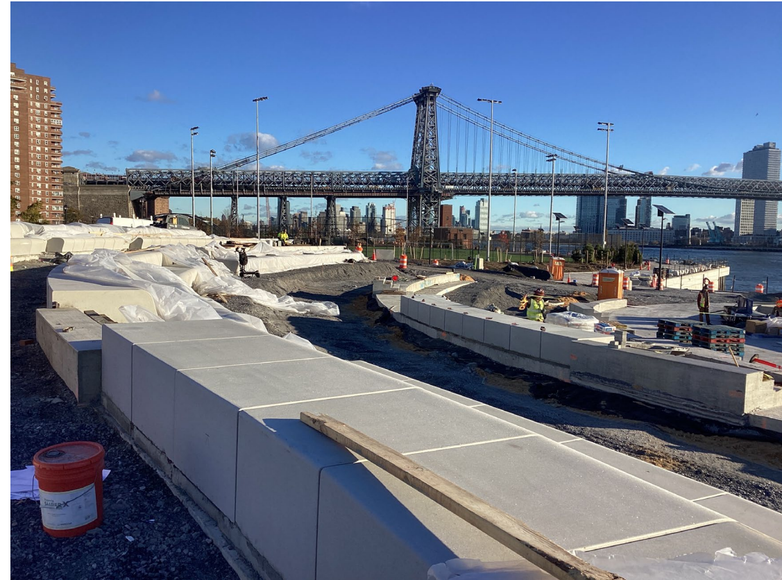
Amphitheater seating installation – November 2024
