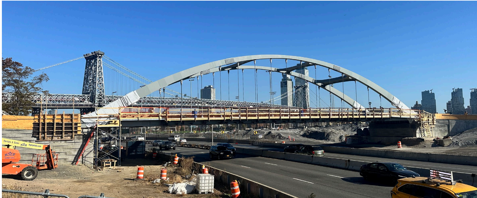
Corlears Hook Pedestrian Bridge installed – November 2024
