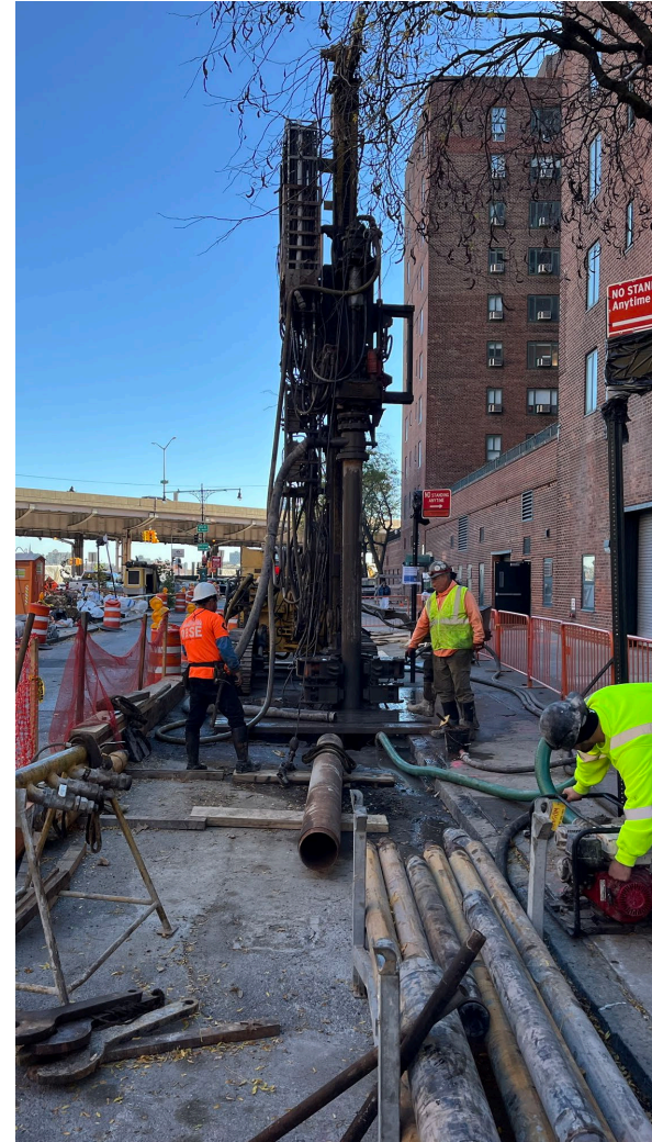
Micropile testing on E. 20 th St. – Nov. 2024
