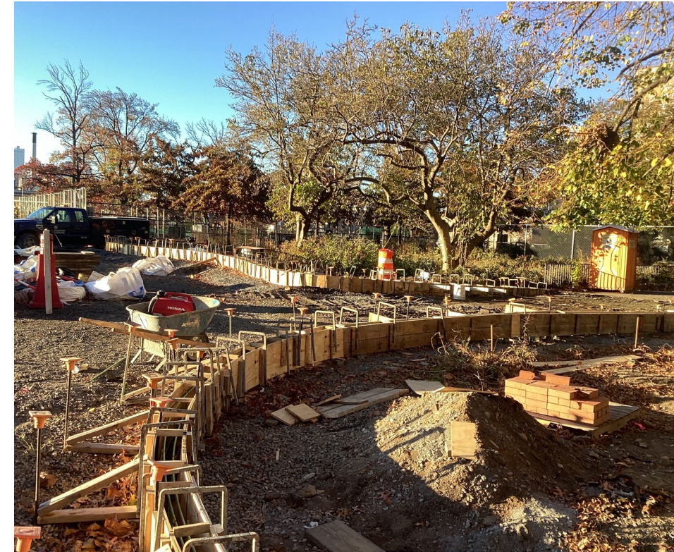
Curb formwork in Corlears Hook Park – November 2024
