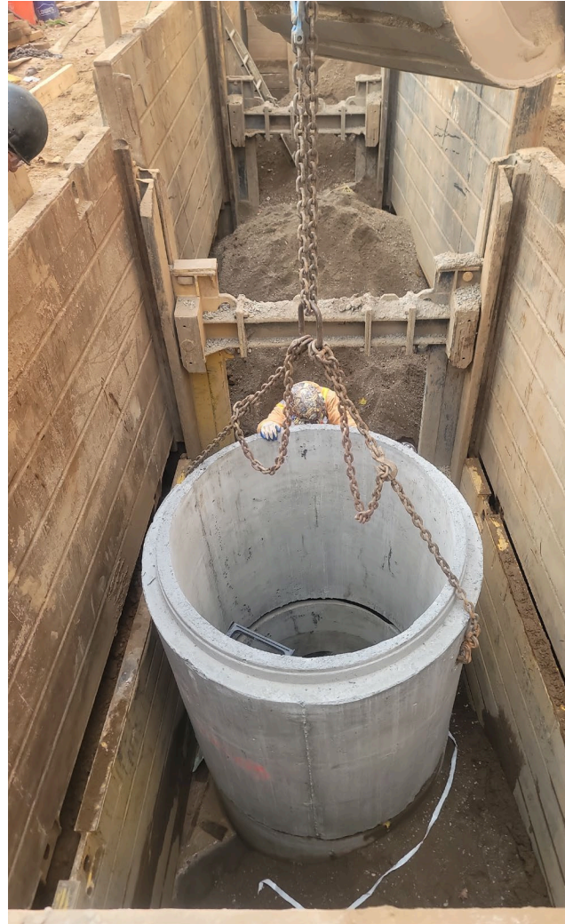
Manhole installation on Water Street – Oct. 2024
