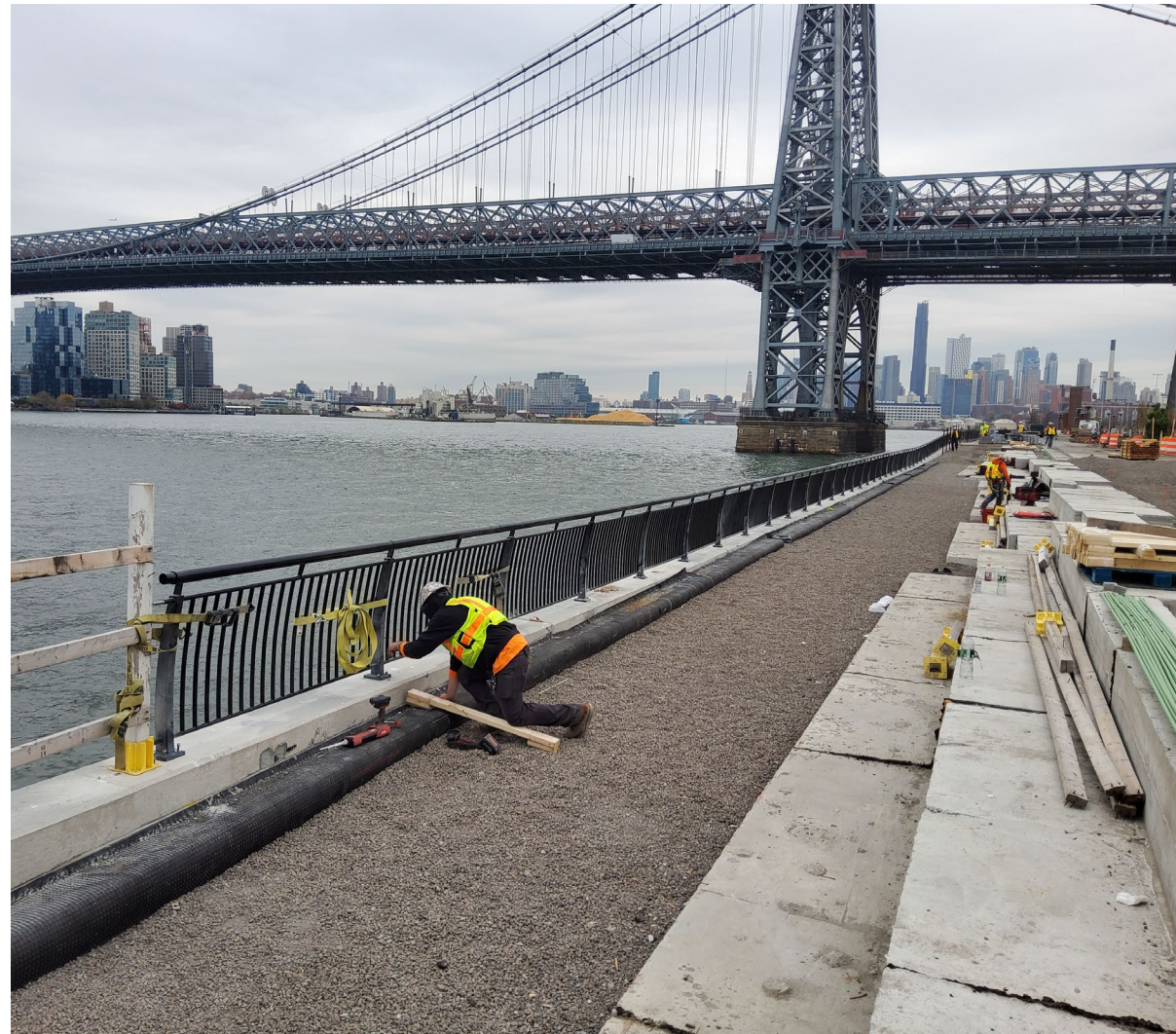
Installation of sea rail along esplanade near Tennis stepdown – November 2024
