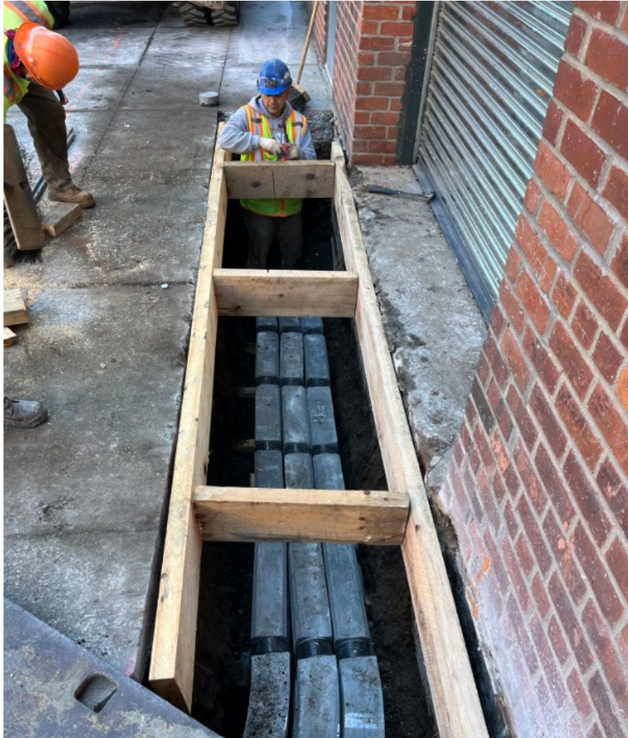
Con Ed conduit installation at E. 20 th Street – November 2024
