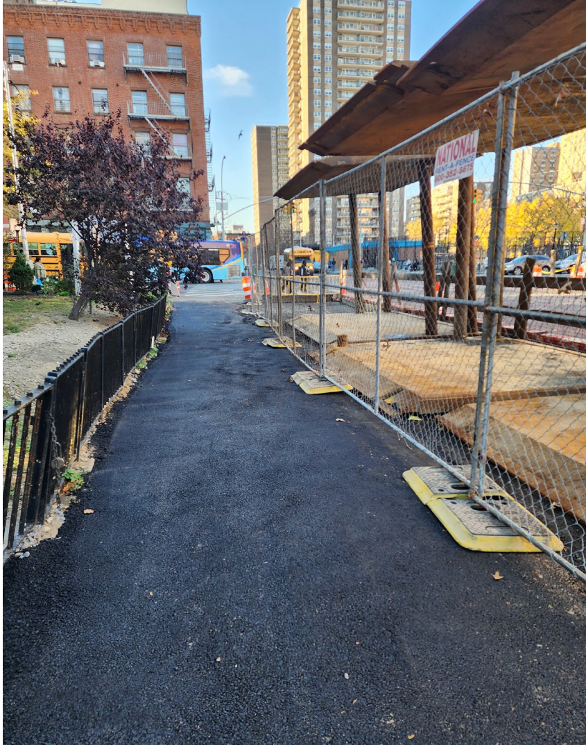
Pedestrian pathway on E. 10 th Street (looking towards Ave D) – November 2024
