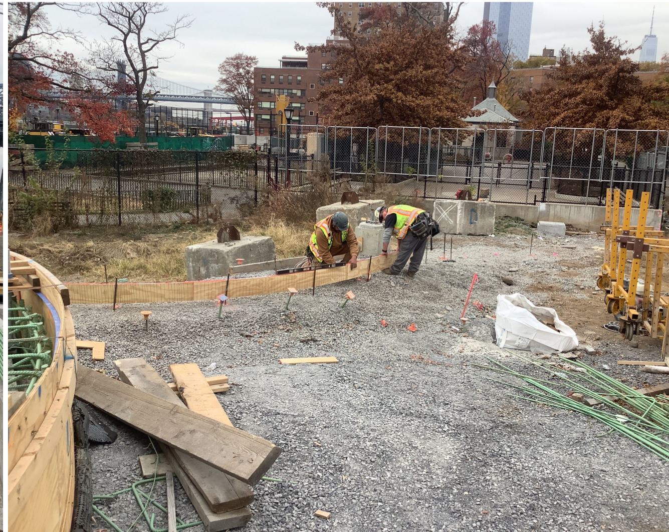
Curb formwork in Corlears Hook Park – November 2024
