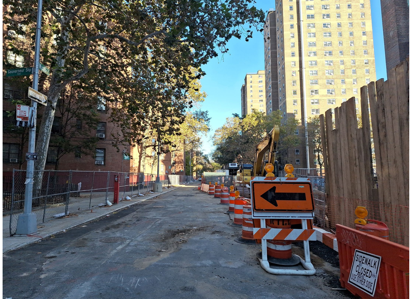
Water St. reopened after completion of deep sewer work – November 2024
