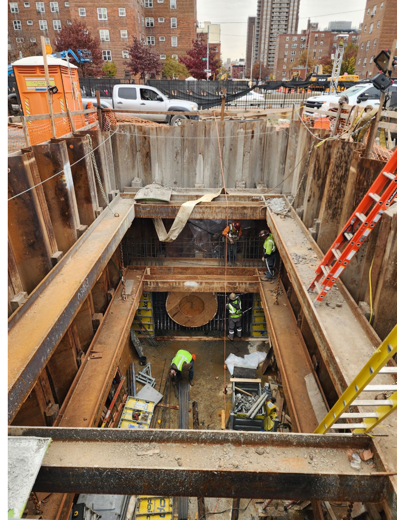
E. 10 th Street microtunneling launching pit – November 2024
