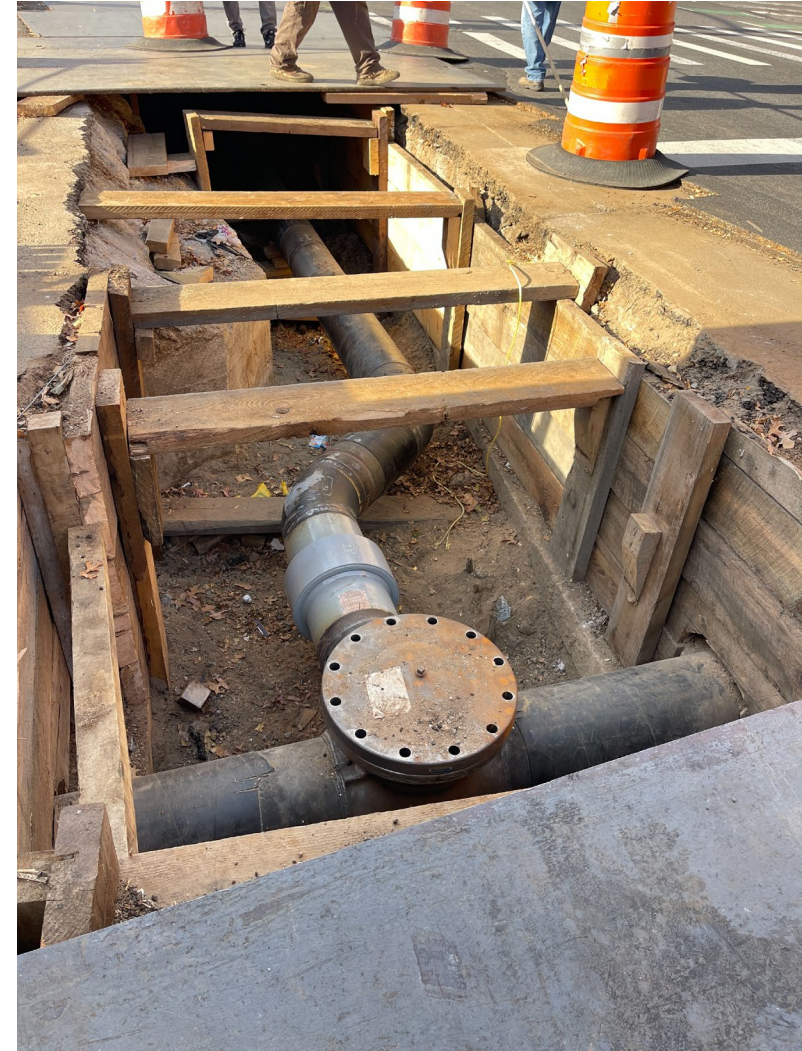
Gas main installation at Columbia St. – November 2024
