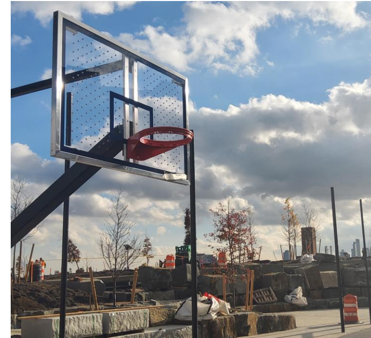
Basketball hoops installed – November 2024
