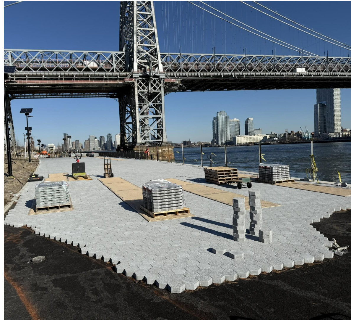
Esplanade paver installation – December 2024
