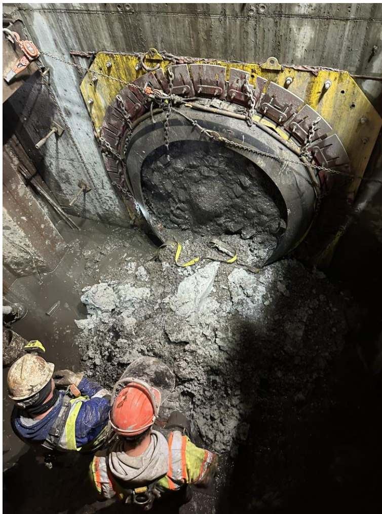
Microtunneling machine breaking through receiving pit – December 12, 2024
