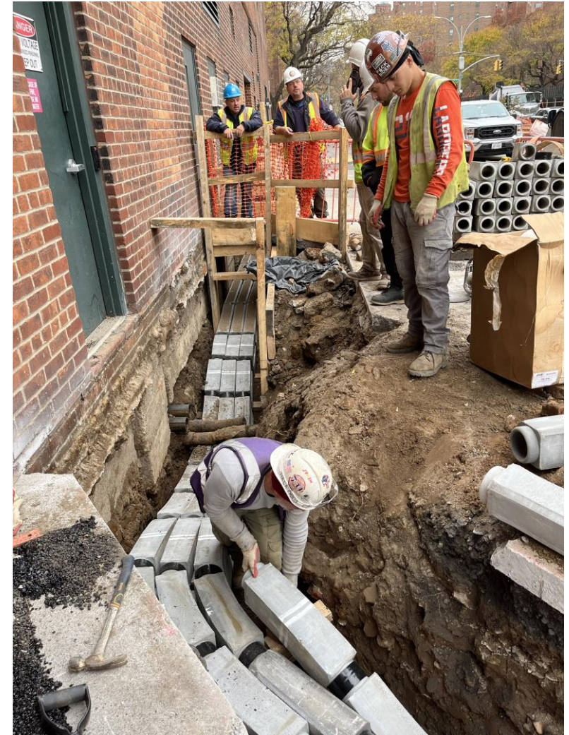
Conduit installation at E. 20 th Street – December 2024
