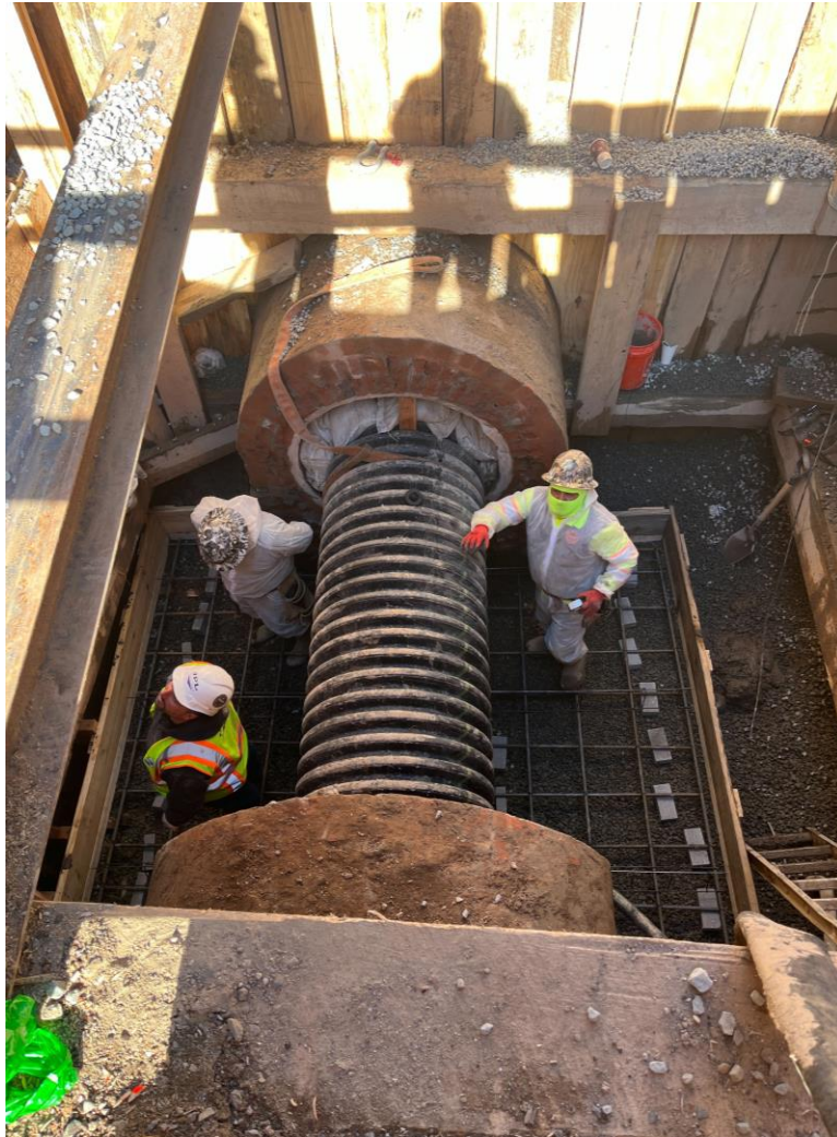
Construction of sewer chamber in Gouverneur Slip E – December 2024
