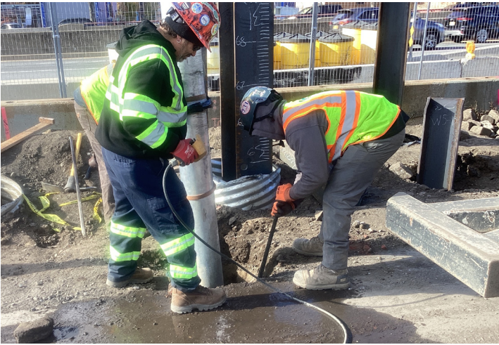
Crews excavating for test pit (PA1), November 2023
