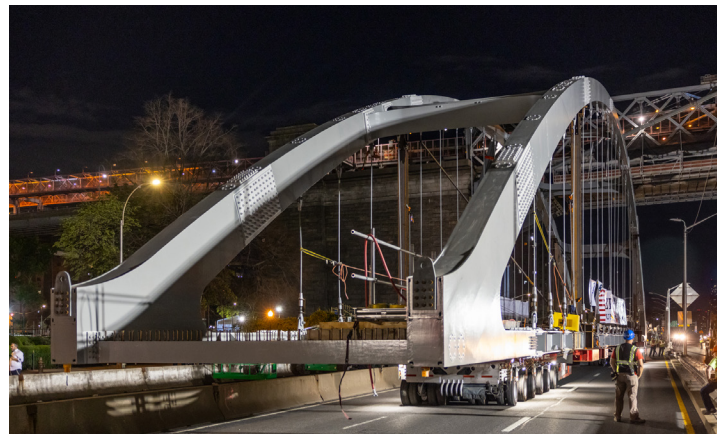
Delancey Street Pedestrian Bridge being rolled on the FDR Drive, June 2024
