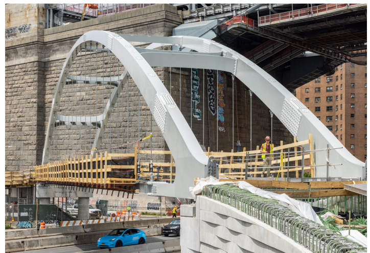
Delancey Street Pedestrian Bridge installed, June 2024
