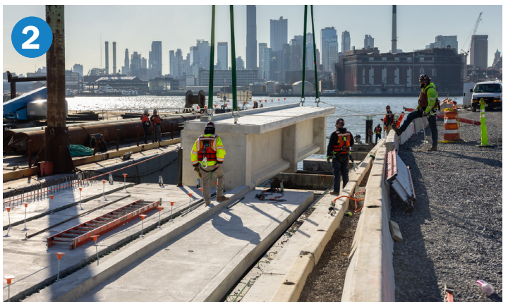
Placing prefabricated esplanade support beams
