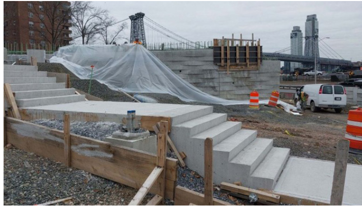
Corlears Hook Bridge western abutment and stairs, March 2024
