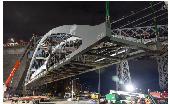
Delancey Street Pedestrian Bridge installation, June 2024
