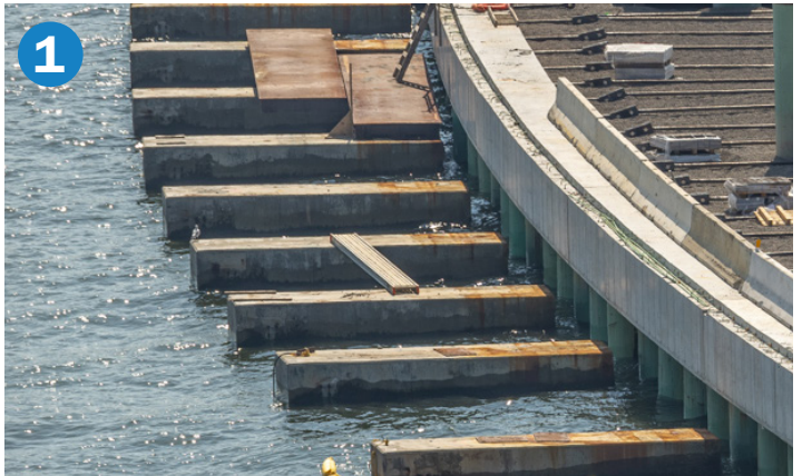
Existing pier caps
