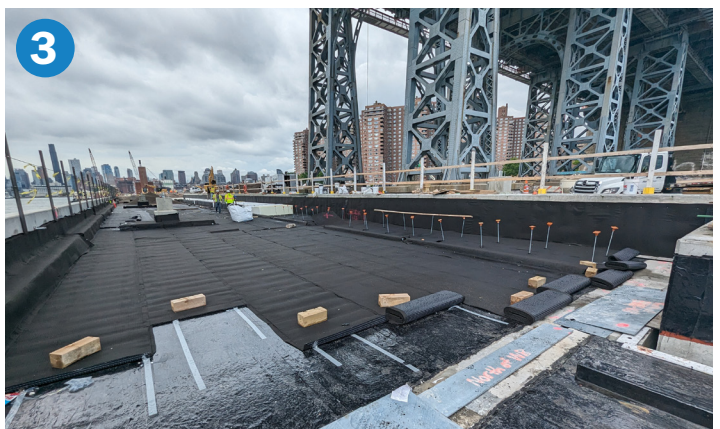
Installation of water-proofing membrane and drainage board
