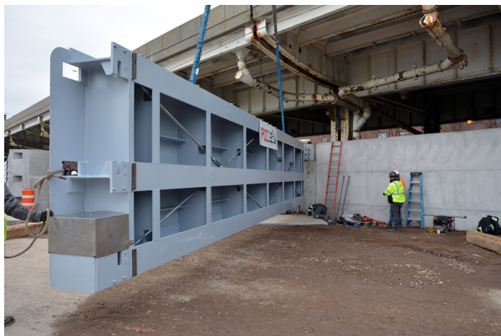
Stuyvesant Cove Park Vehicular Swing Gate install 2/24/2022
