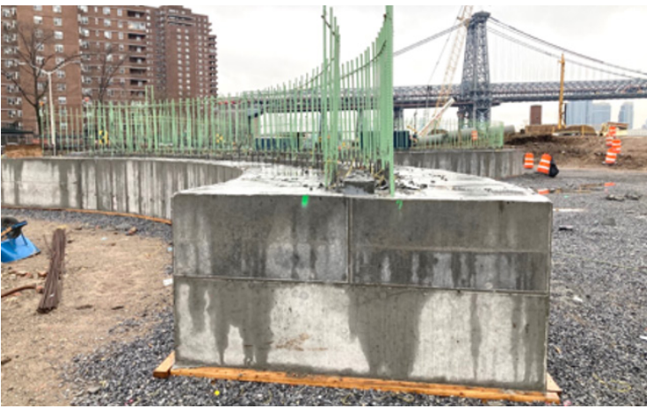
Corlears Hook Bridge East Abutment, January 2023
