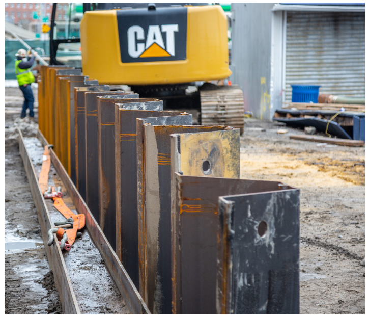
Sheet pile installation in Stuyvesant Cove Park
