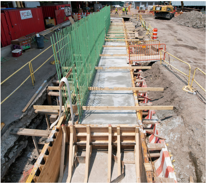
Foundation and formwork for the first section of floodwall in Stuyvesant Cove Park.
