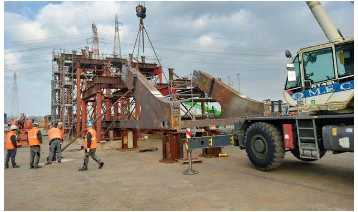
Test fit of Delancey Street Bridge at fabrication facility, November 2023
