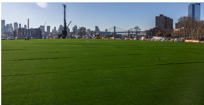
Synthetic turf being placed on Ballfields 1 and 2, December 2023
