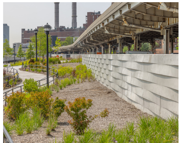
Plantings and floodwall in Stuyvesant Cove Park, 2023
