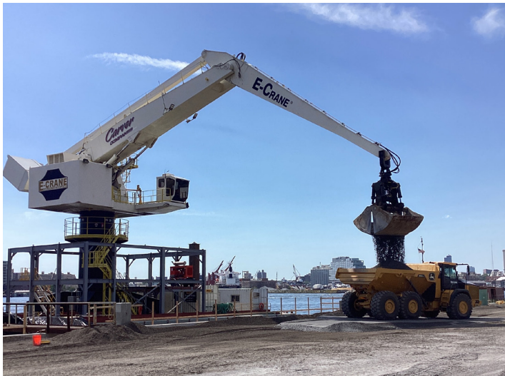
Crane unloading fill materials from barge, September 2023
