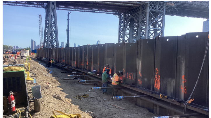
Floodwall to be buried near esplanade and Williamsburg Bridge, August 2023
