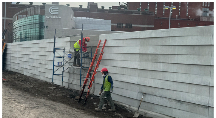
Floodwall work south of Murphy Brothers Playground, December 2023
