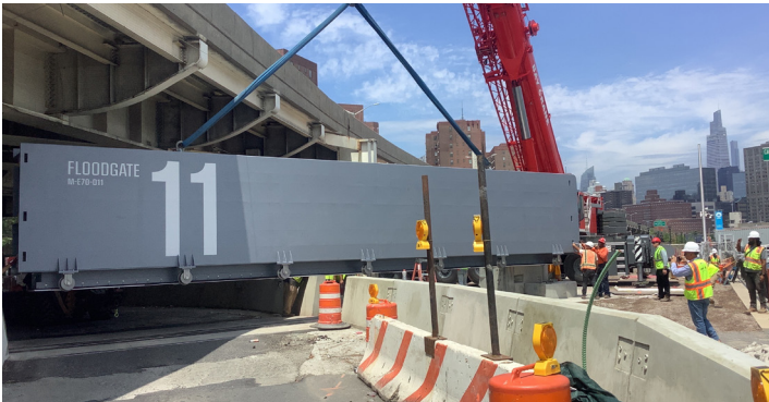
Installation of Floodgate 11, July 2023
