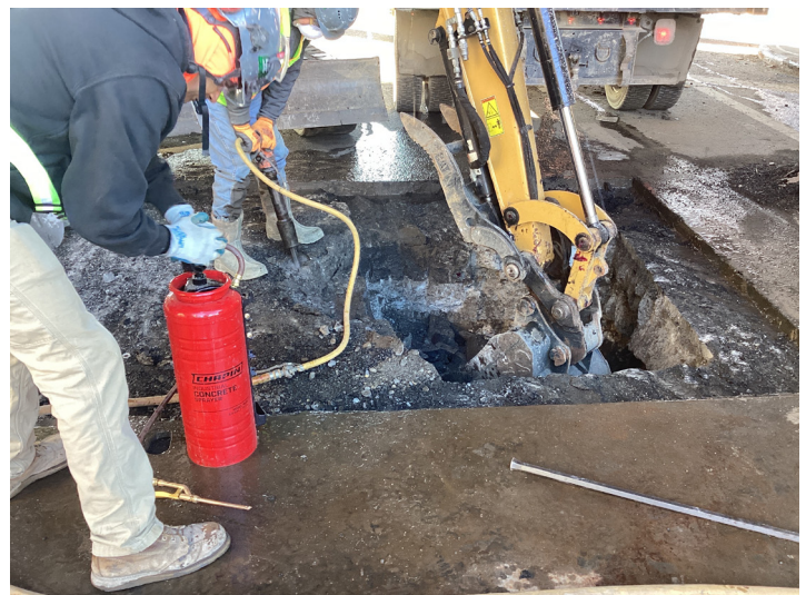
Test pit excavation to locate ConEd utility ducts (PA1), November 2023
