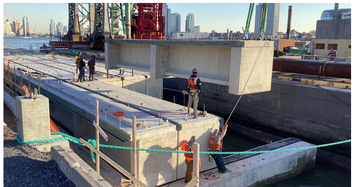
Installation of pre-cast esplanade pieces, December 2023
