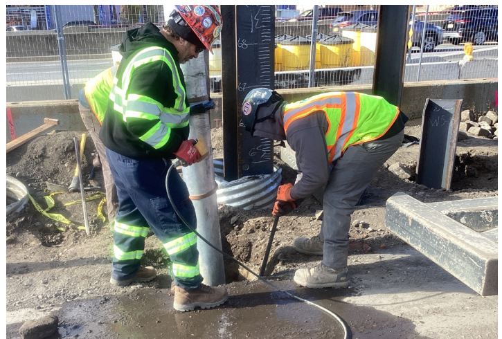
Crews excavating for test pit (PA1), November 2023
