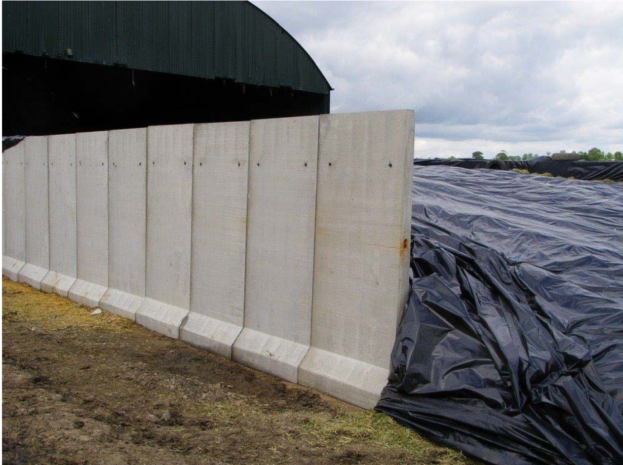
Precast concrete wall
