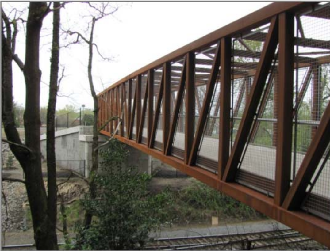
Typical prefabricated pedestrian bridge (124 ft long, 14 ft wide)
