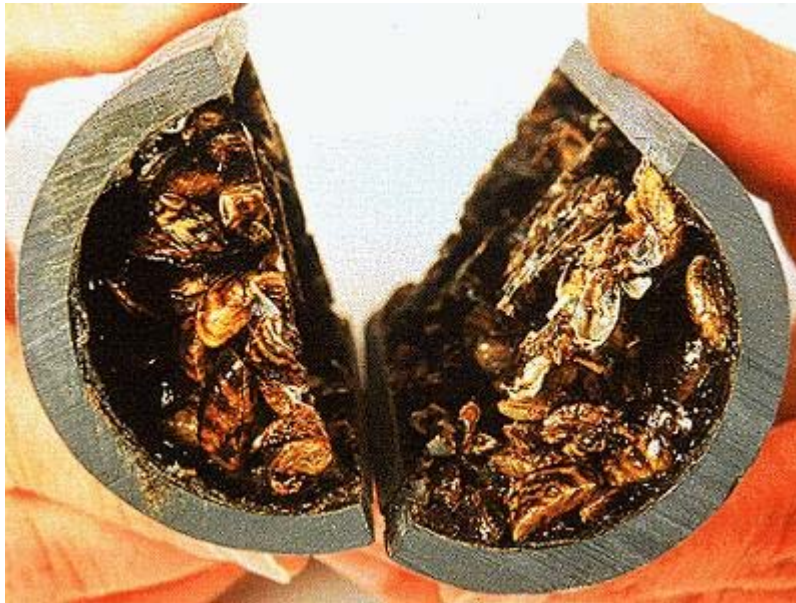
Piping Infested with Zebra Mussels
