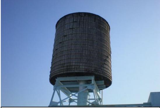
**AN EXAMPLE OF A TYPICAL GRAVITY TANK**
