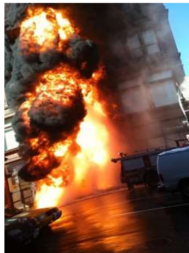
Transformer Fire (Note height of the flames in relation to FD engine)
