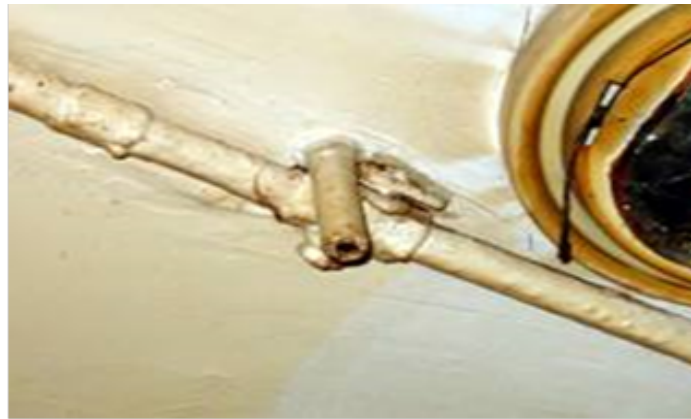
Old gas line for lighting run along the ceiling
