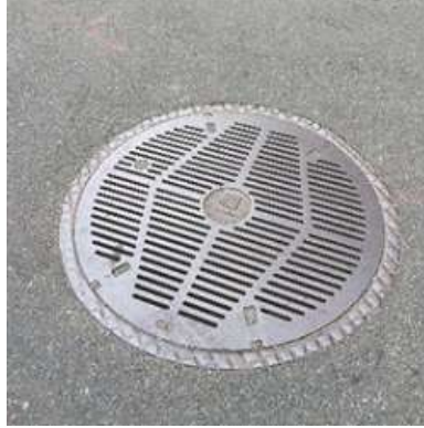
Vented Manhole Cover
