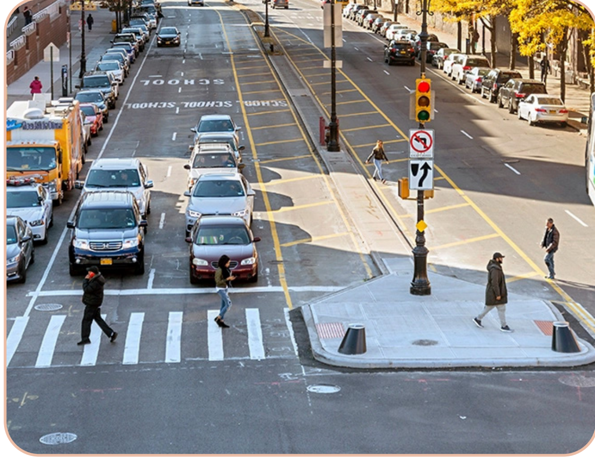
A "road diet" or lane narrowing and lane removal (Grand Concourse and E 149th Street, Bronx)
