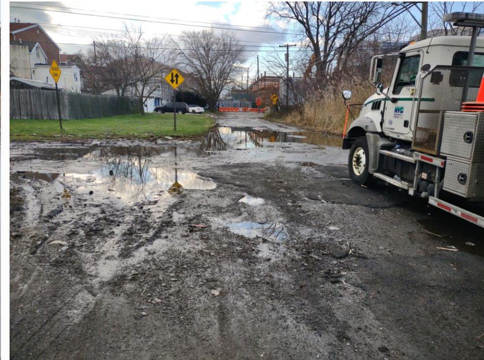
Drier conditions on Sapphire Street after DEP pumping.
