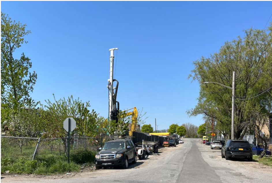
Construction happening across from residences in the Jewel Streets.
