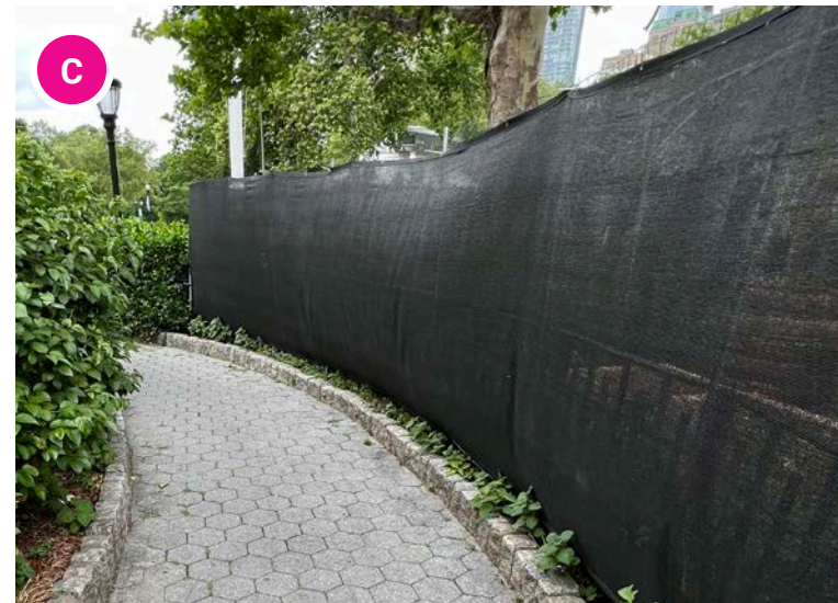
8' screening along 3' steel fence
