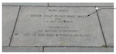
GRANITE PAVER TO HAVE ENGRAVED TEXT AT 1/4" DEPTH MAX. TEXT TO MATCH EXISTING IN STYLE AND SIZE:
