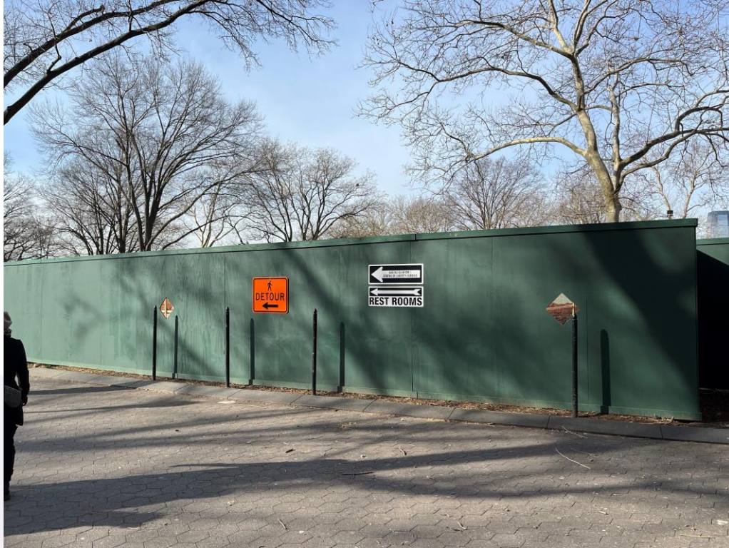
Construction Fence Installation In Progress
