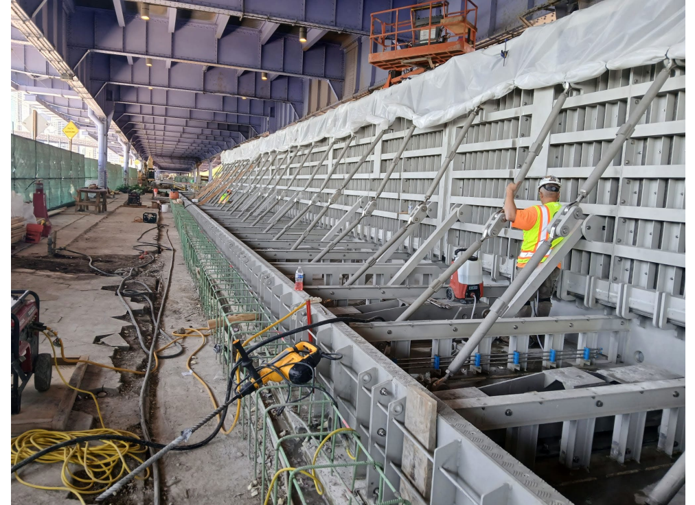
Deployed flip up gate during installation – June 2024
