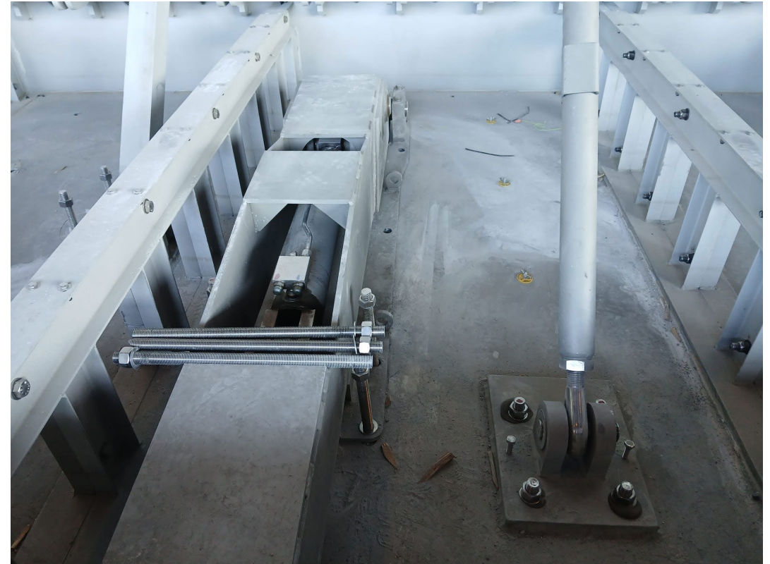
Flip up gate hydraulics – June 2024
