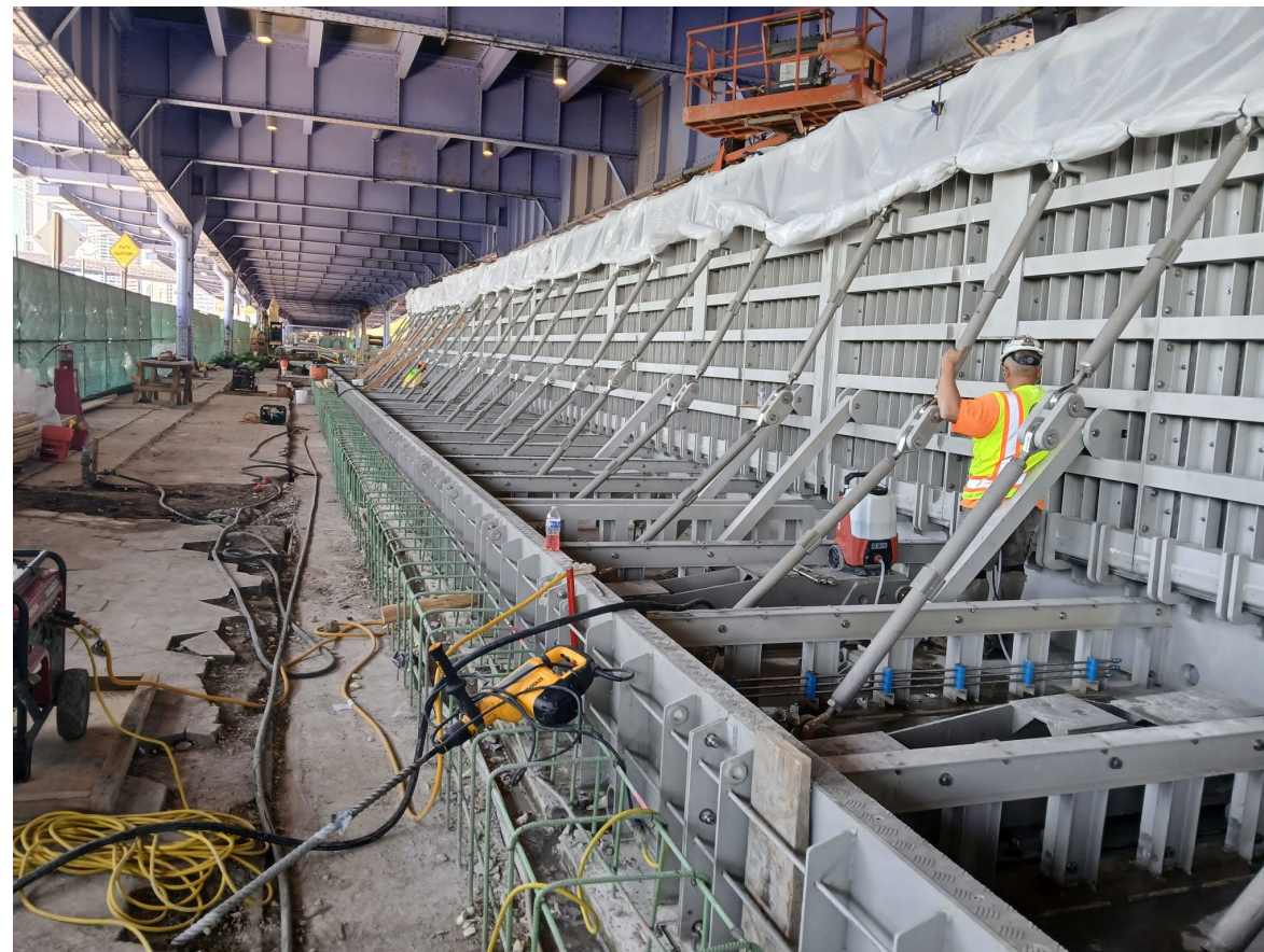
Deployed flip up gate during installation - June 2024
