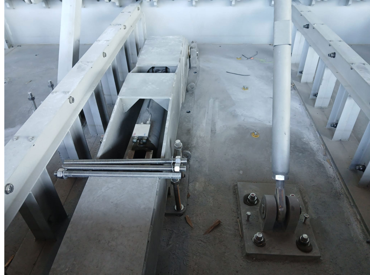
Flip up gate hydraulics – June 2024
