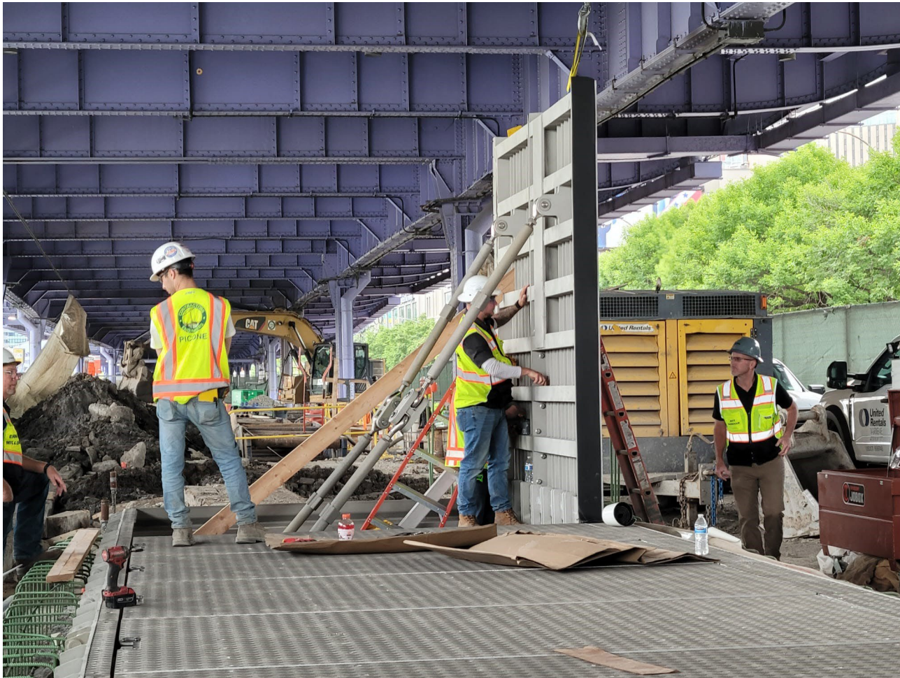
Contractor bolting flip up gate segments together – June 2024
