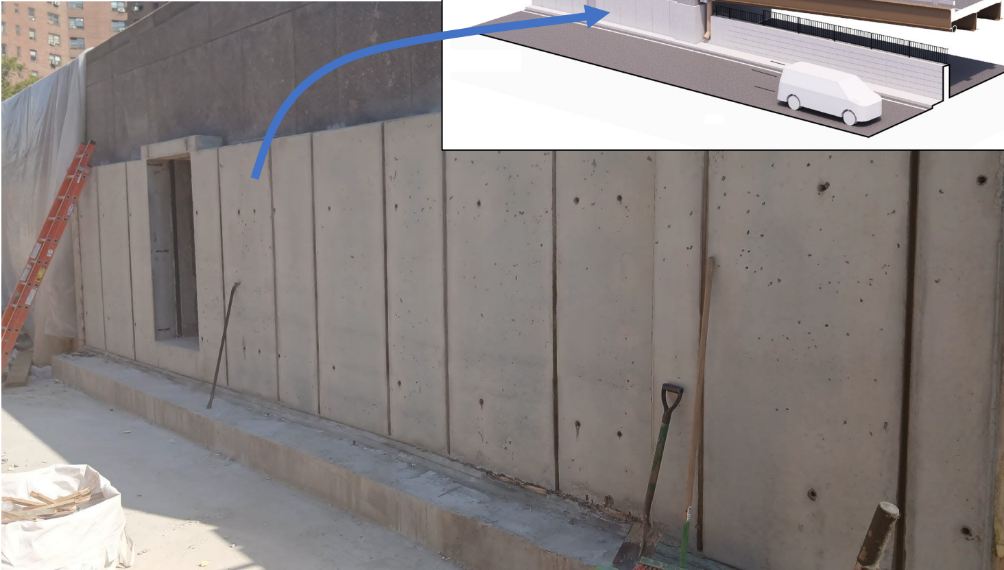
Floodwall tie-in to FDR Drive off-ramp – September 2024
