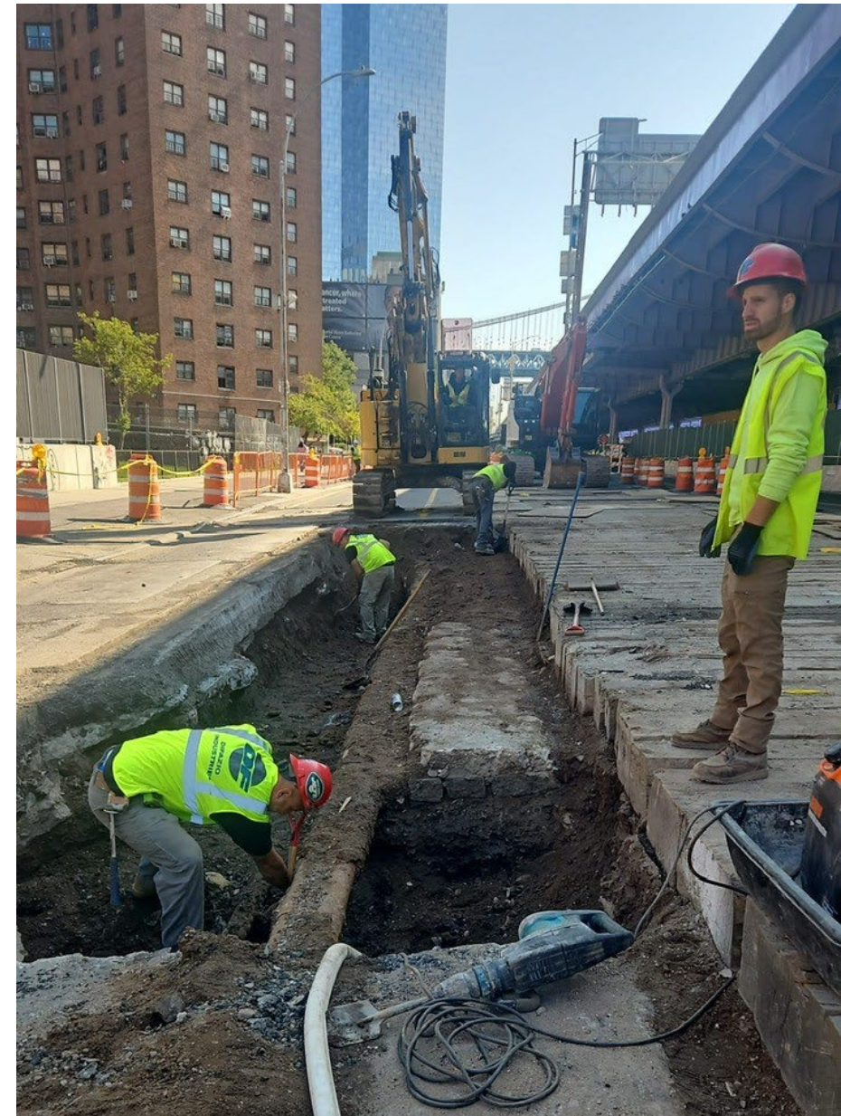
Utility work in South Street – September 2024
