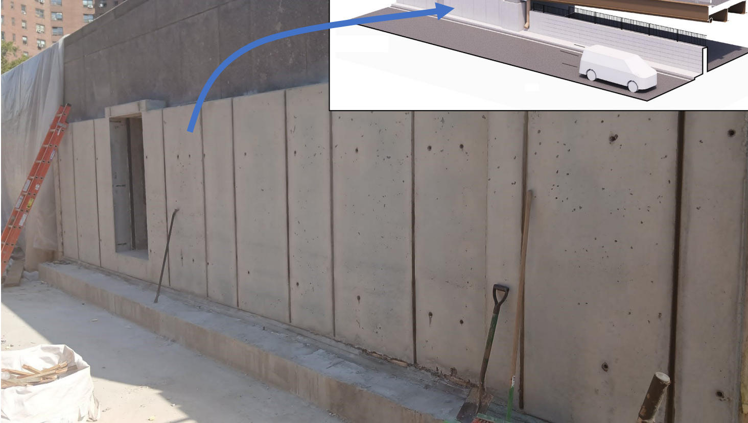
Floodwall tie-in to FDR Drive off-ramp – September 2024
