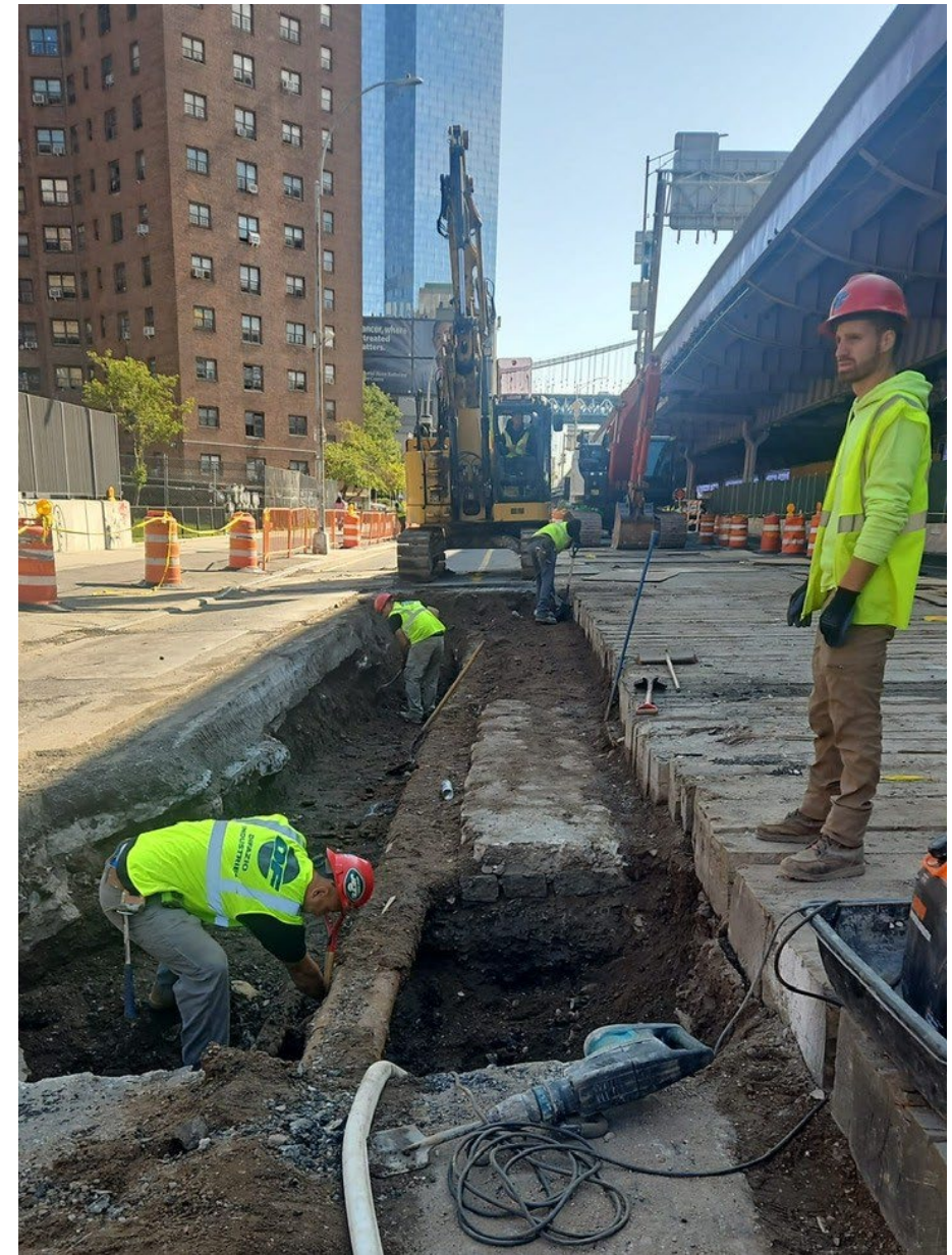
Utility work in South Street – September 2024
