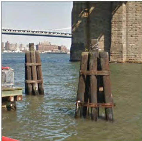
Wooden Pier Pillars
