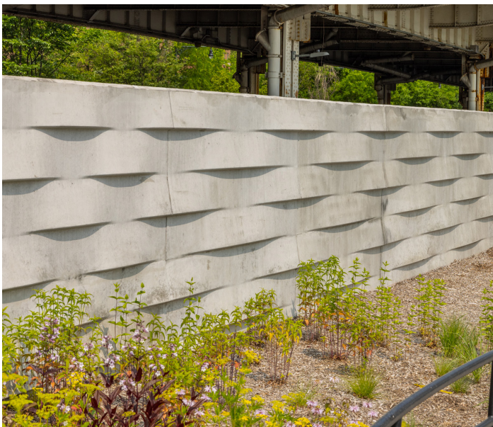
Wave pattern of floodwall in Stuyvesant Cove Park, May 2023
