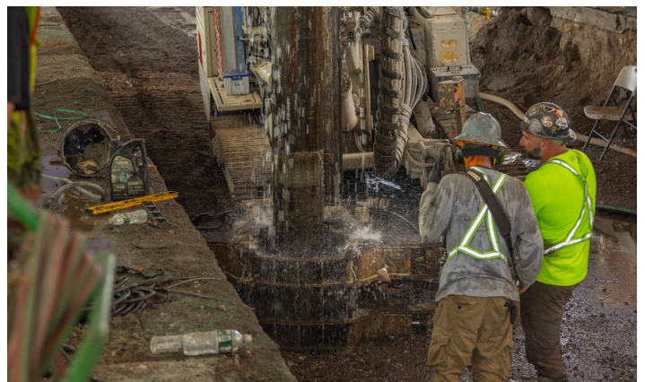
Micropile being drilled into ground, September 2023
