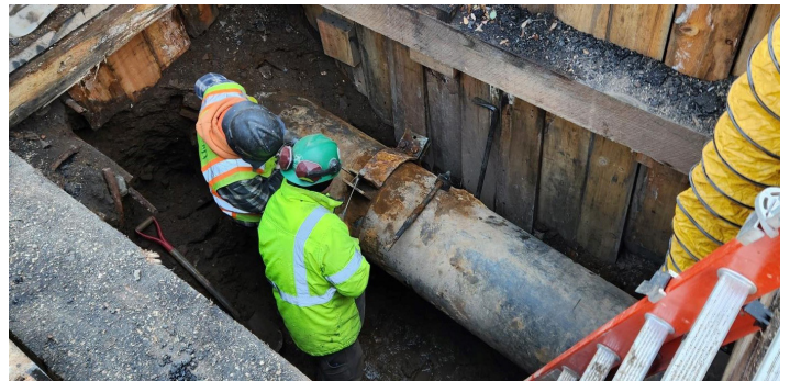
20-inch water main installation, November 2023
