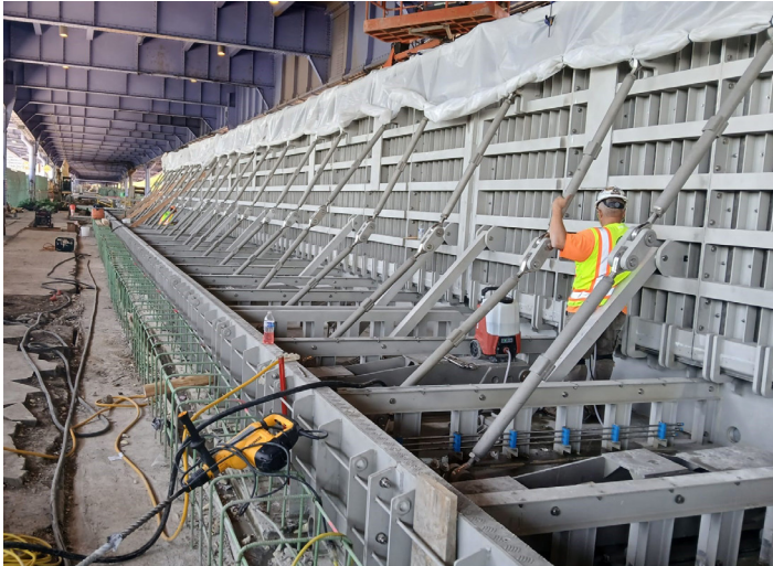
Flip up gates being installed, June 2024
